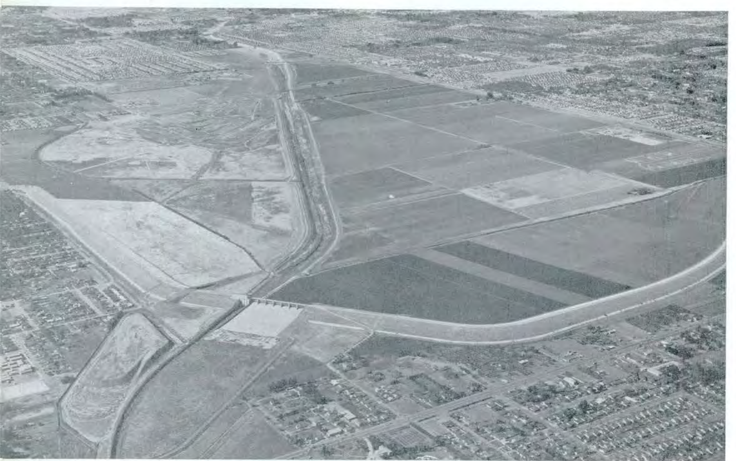
South Coastal Area—Morris Dam on San Gabriel River (top), and Sepulveda Flood Control Reservoir on Los Angeles River
