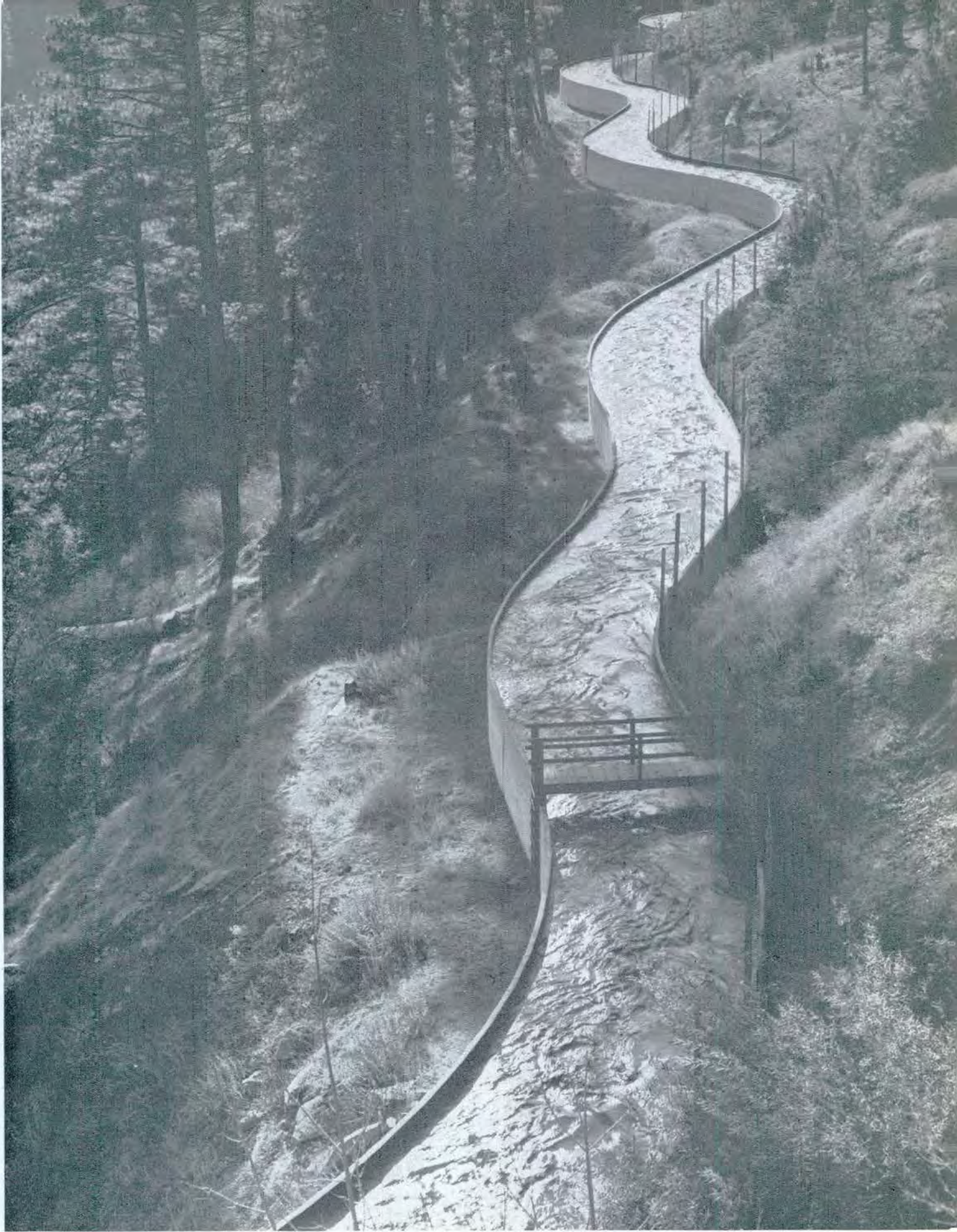
San Joaquin River Basin—Diversion Flume From Mokelumne River
