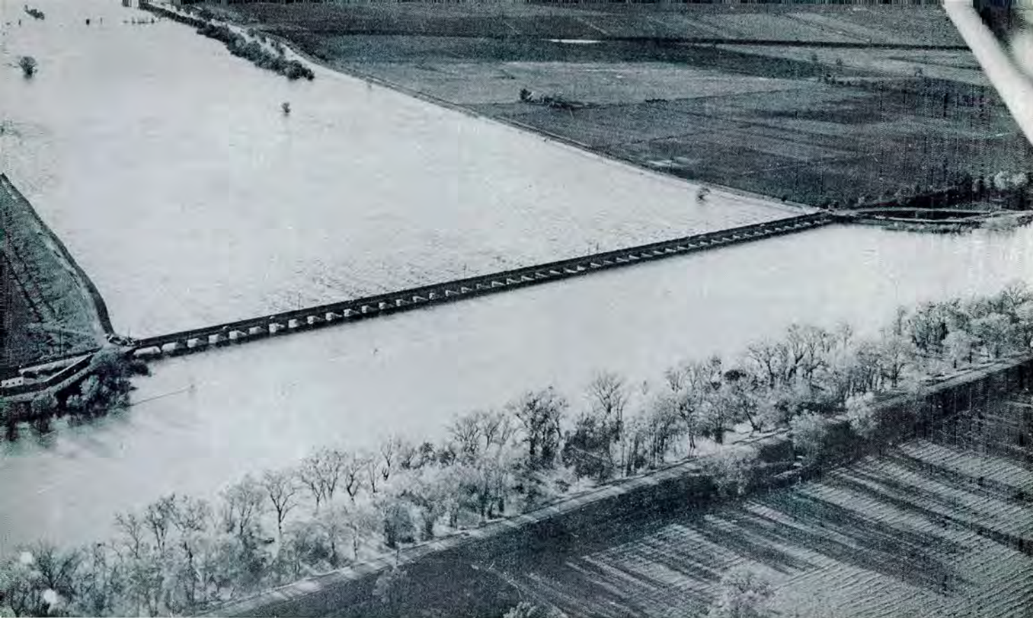
"Generally, it is not feasible to attain . . . flood control by storage alone." Sacramento Weir on Sacramento River
