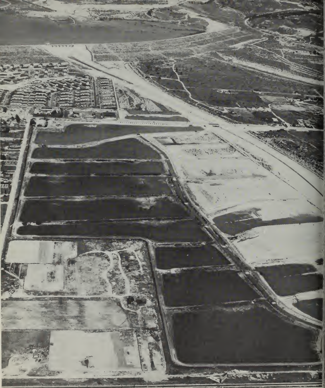
"Storage of water underground through artificial recharge has been widely practiced in California since 1895." Hansen Spreading Grounds Near Burbank
