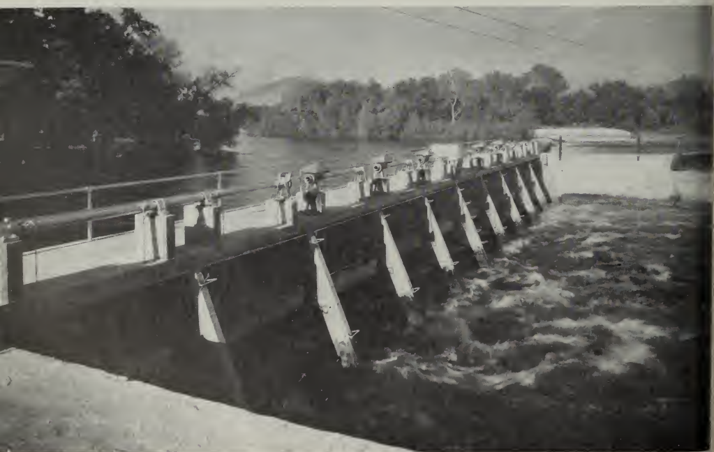
Diversion Dam and Irrigation Canal Headgates on Kings River
