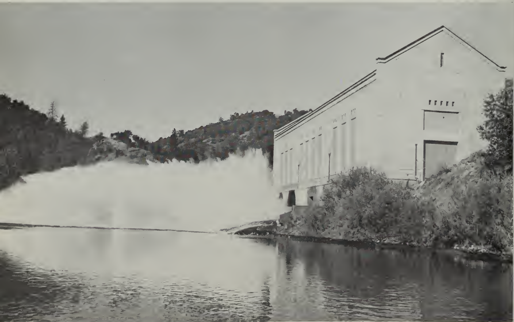
". . . hydroelectric power as an inseparable part and partner in California's water resource development is a fully recognized requisite . . ." Elverta Power Plant on Mokelumne River
