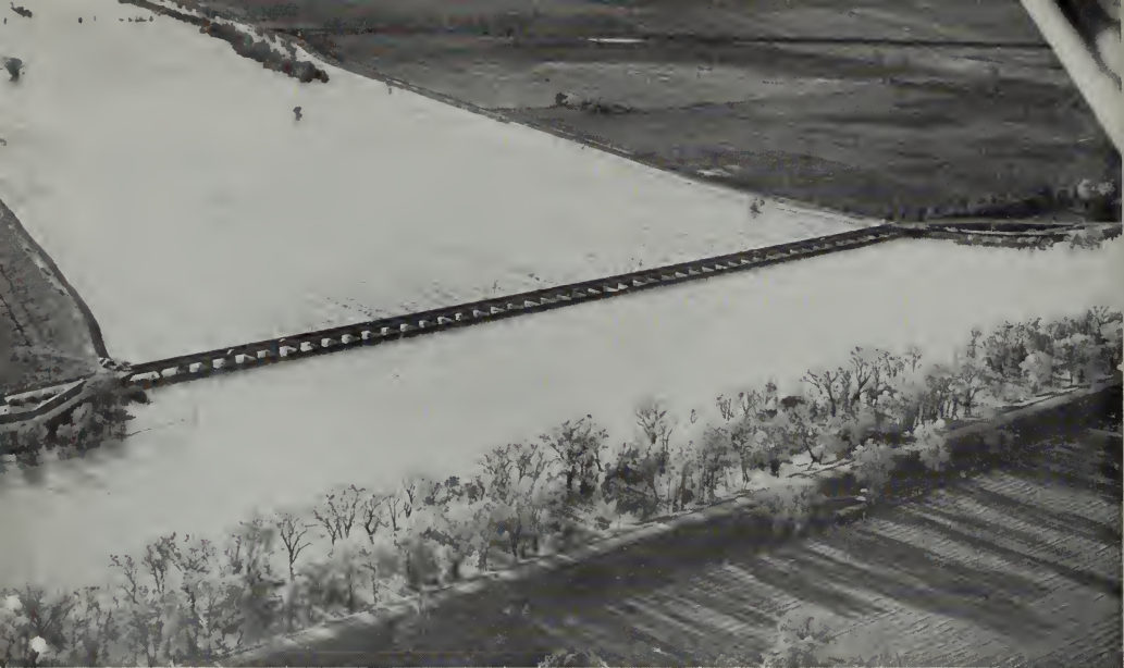
"Generally, it is not feasible to attain . . . flood control by storage alone." Sacramento Weir on Sacramento River
