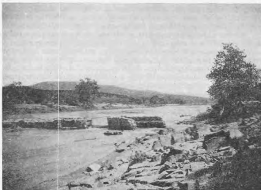
MISSION DAM ON SAN DIEGO RIVER
