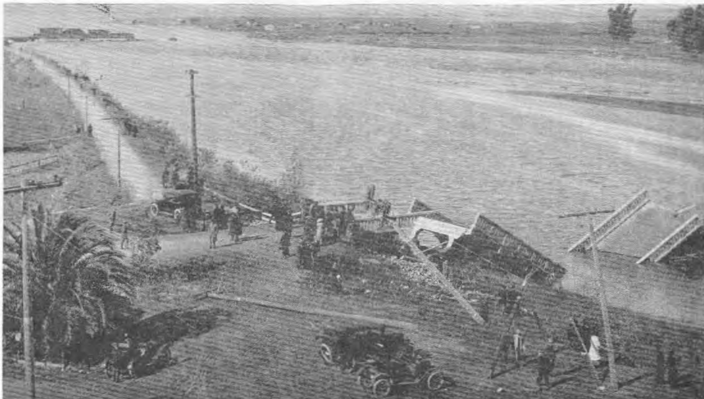
FLOOD DAMAGE ALONG SAN DIEGO RIVER—1915
