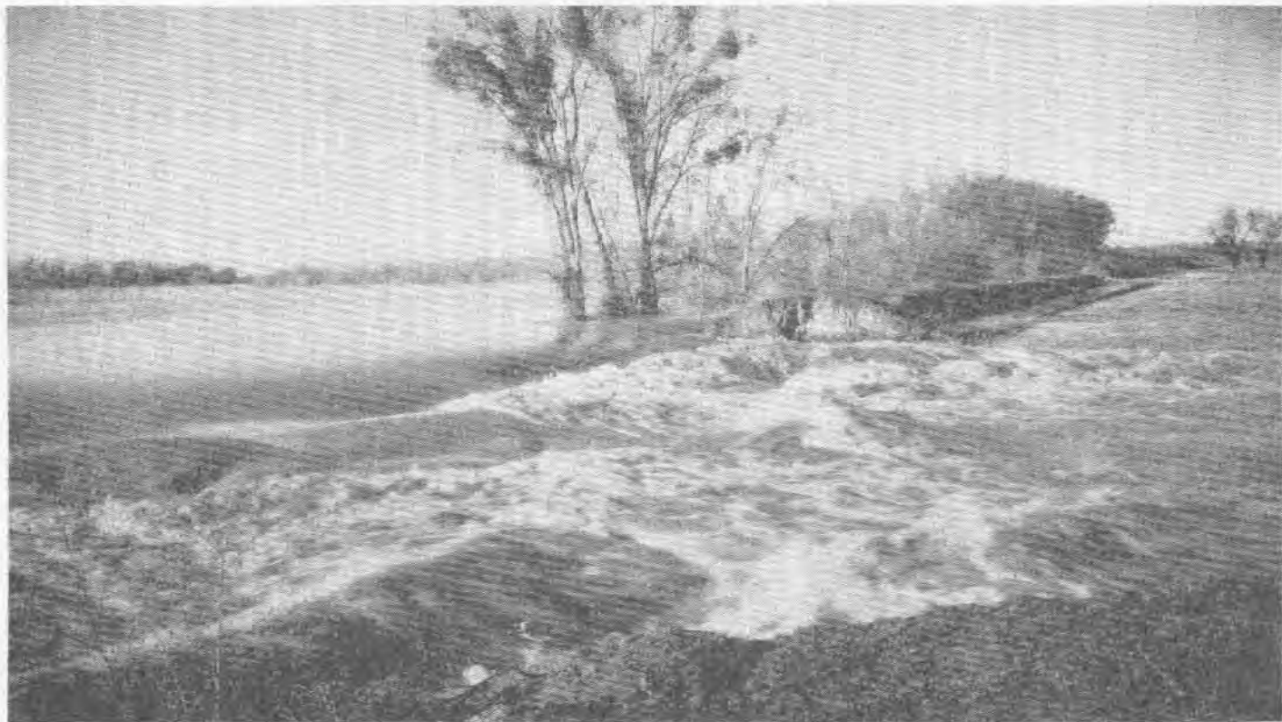
BREAK IN SACRAMENTO RIVER LEVEE DURING 1936 FLOOD
