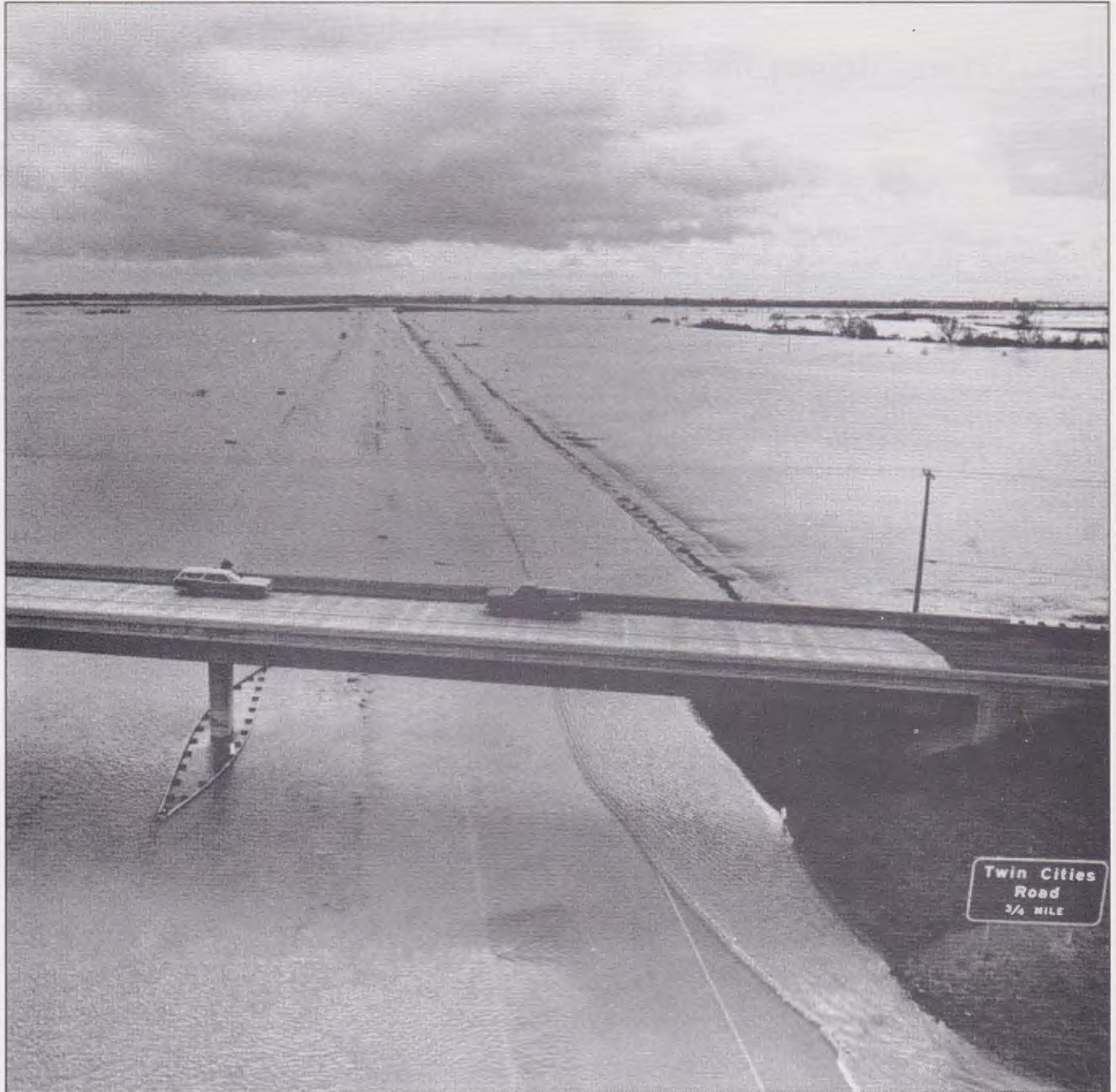
During the February 1986 storms, Interstate 5 was closed for about 2 weeks in the Walnut Grove-Thornton area because of the flooding.
