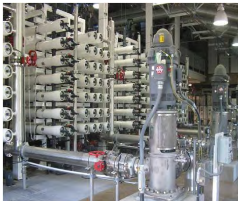
Reverse osmosis treatment is one step in the purification process that makes recycled water suitable for potable purposes
