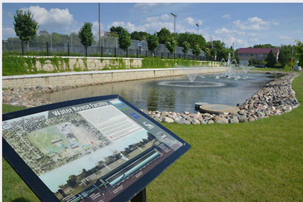
FIGURE 1-3-1 A half million-gallon stormwater storage reservoir at Saint Anthony Village lies below an attractive stormwater pond with fountains. The system reduces the use of water treated to drinking water standards for irrigation and reduces phosphorus discharges to surface water. SOURCE: Metropolitan Council (2011).
