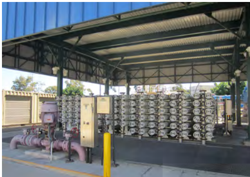
Terminal Island Water Reclamation Plant
