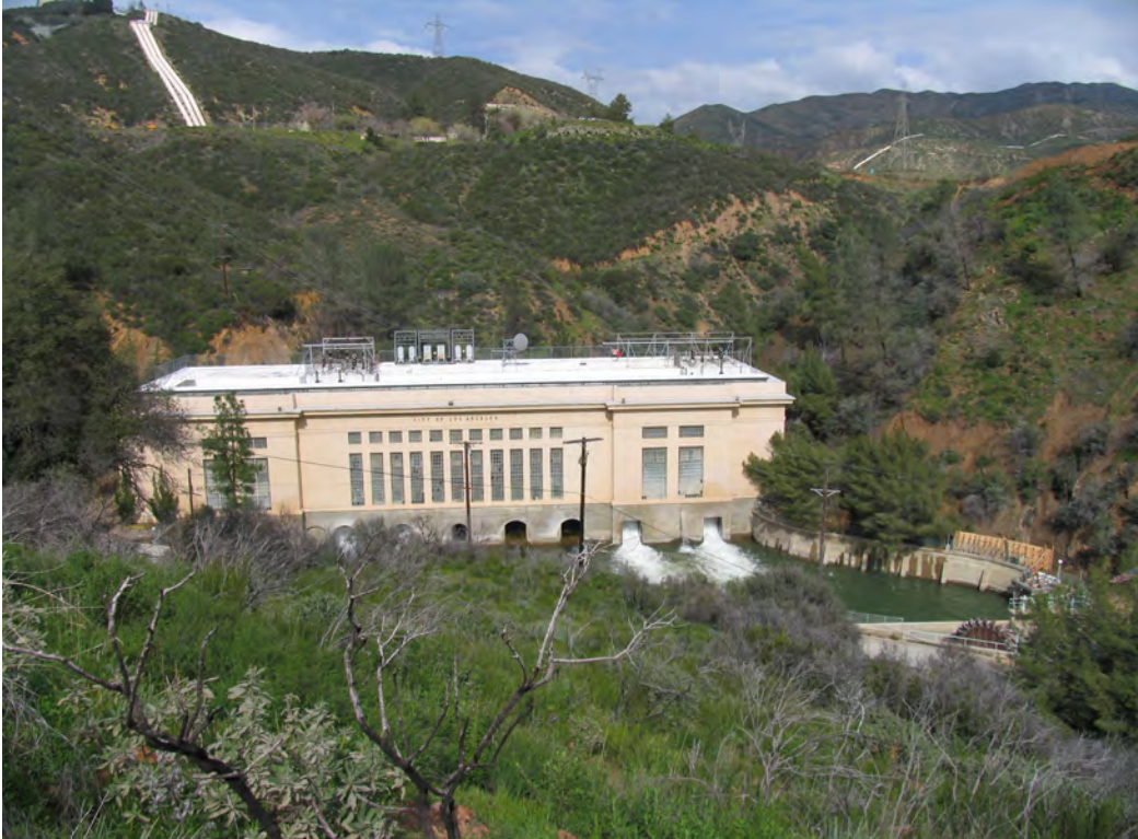
San Francisquito Power Plant Number 1
