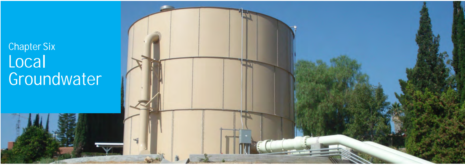
Mission Wellfield Water Tank
