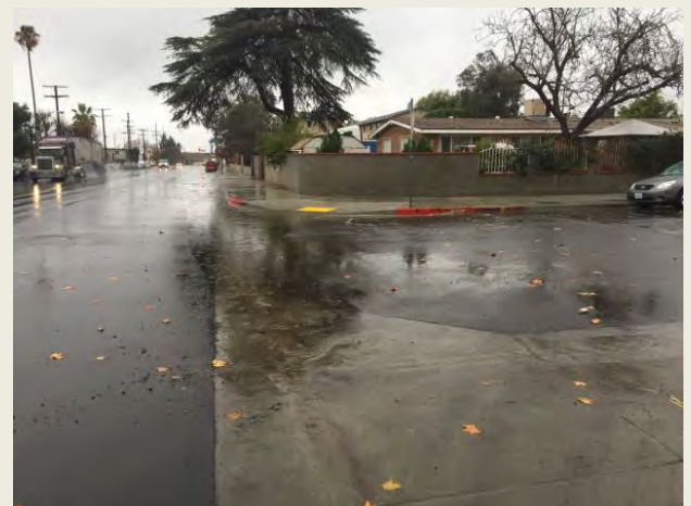
Intersection After Construction
