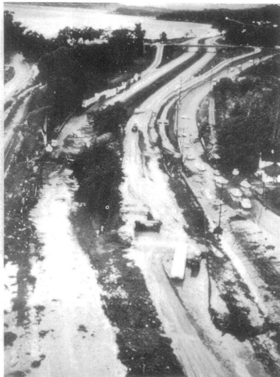
Figure 19 — View of Highway 101 and Southern Pacific Railroad flooded by overflow from Toro Canyon Creek during December 1971. (Note trucks jack-knifed on highway.) Both railroad and the highway were out of service for many hours.
