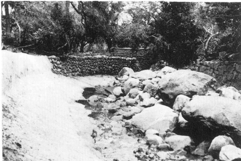
Figure 11 -- Montecito Creek, near Hot Springs Road, after November 1964 flood. Large boulders carried by the flow were deposited upstream from the bridge.
