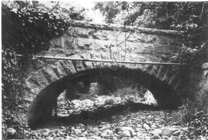
Figure 2 — Romona Lane bridge over Oak Creek (looking upstream at river mile 0.54).
