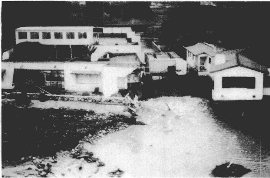
Figure 14 — Oak Creek, at the ocean, eroded its banks and undercut existing structures during January 1969 flood.
