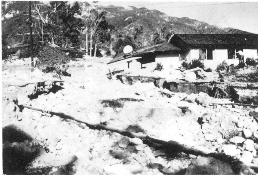
Figure 17 -- Romero Canyon Creek, near Featherhill Road, after January 1969 flood. Boulders, carried by the flow, crashed through this home and others.
