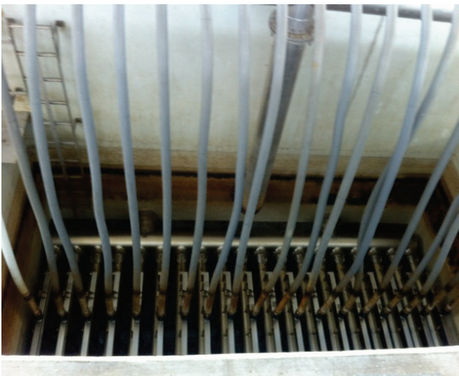
Figure 6-2. Submerged MF membranes at OCGWR
