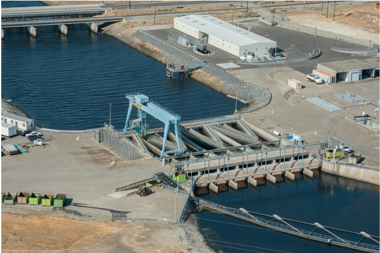
Figure 4-4 Skinner Delta Fish Protection Facility
