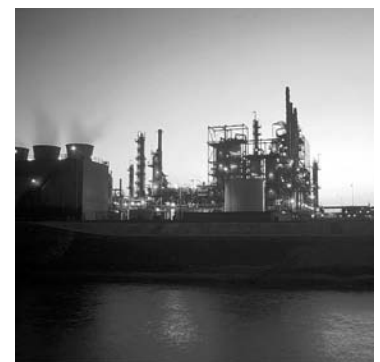
West Basin Municipal Water District delivers recycled water to Chevron Oil Refinery in El Segundo, CA., for use in cooling towers.
