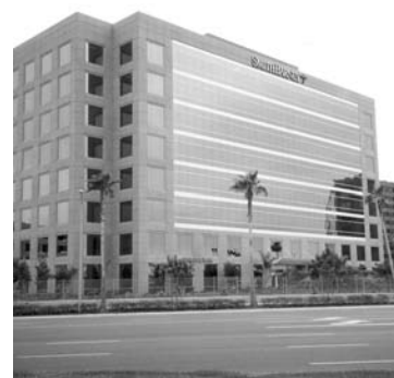
Recycled water is used for toilet and urinal flushing in the recently constructed Smith Barney building in Irvine, CA.
