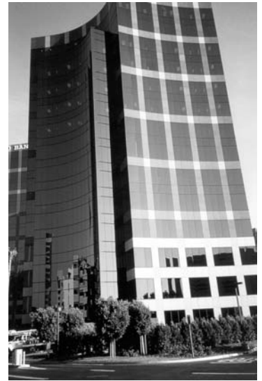
The Opus II building in Irvine, CA, uses recycled water treated by Irvine Ranch Water District in air conditioning cooling and toilet and urinal flushing.
