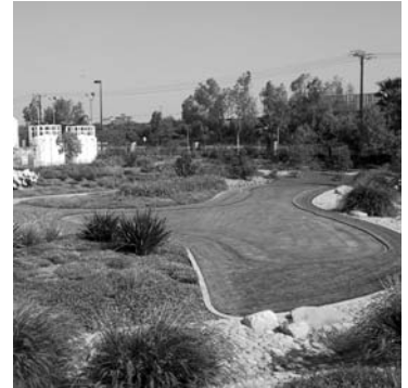
The Inland Empire Utilities Agency's Carbon Canyon Water Recycling Plant provides water (10 mgd) primarily for landscape use in Chino and Chino Hills, CA.
