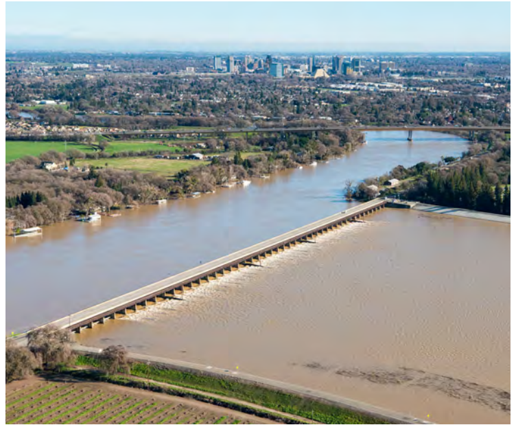
Gates on the Sacramento Weir were opened in 2017 to allow water to flow from the Sacramento River into the Yolo Bypass. The 1,920-foot long weir, constructed in 1916, is one of multiple structures making up the Sacramento River Flood Control Project. Its manually operated gates are opened based on forecasted river flows to reduce Sacramento River flood stages downstream of the American River confluence, to reduce flood risk to the metropolitan Sacramento area. Prior to water year 2017, the gates were last opened in December 2005.
