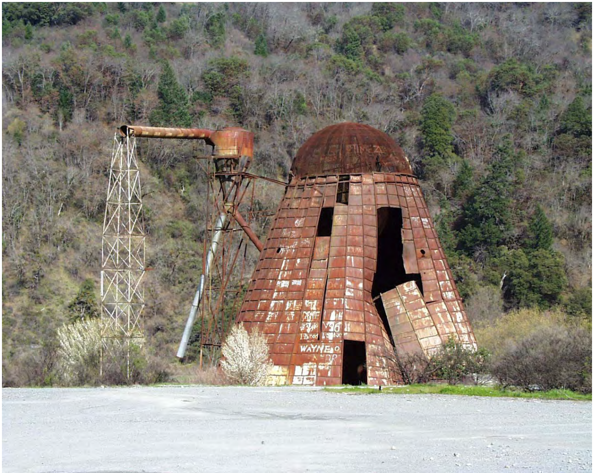
Tee-Pee Burner at Abandoned Cal-Pac Mill (2000)
