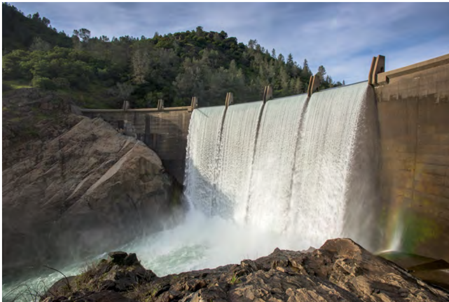
The Lower Lake Clementine Dam on the North Fork American River in Placer County in Northern California. Photo taken March 31, 2016.
