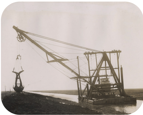
A clamshell dredge uses river-bottom material to form unengineered levees in the Central Valley, circa 1910–1930.
