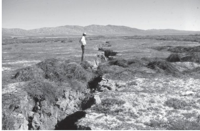
Figure 11. Earth fissure associated with land subsidence caused by groundwater pumping in Fremont Valley, California, March 1978 (from Holzer and Galloway, 2005).
