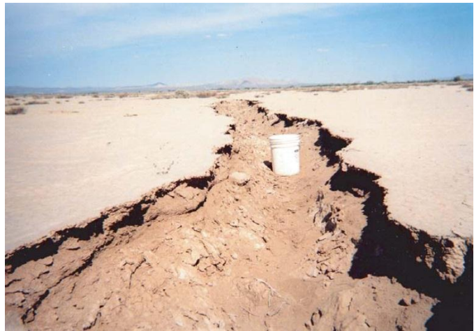
Figure 12. Earth fissure near the southeast edge of Lucerne Lake playa in the Mojave Desert, California. View is to the northeast, with a five-gallon bucket for scale. (Sneed et al., 2003a, Fig. 6 B)
