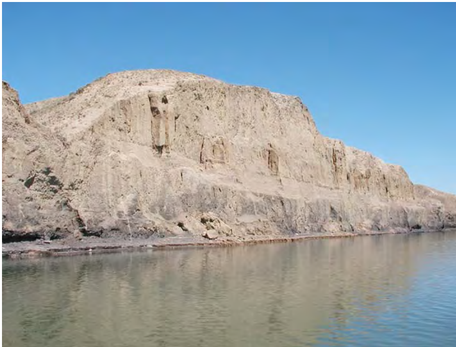
Figure 9.5. Eroded bank material depositing below the water line (photo by S. Nuanes).
