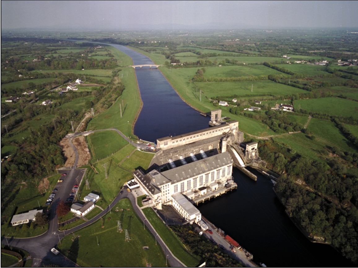
Figure 201. Aerial view of Ardnacrusha hydroelectric power plant in Ireland. (Courtesy of ESB)
