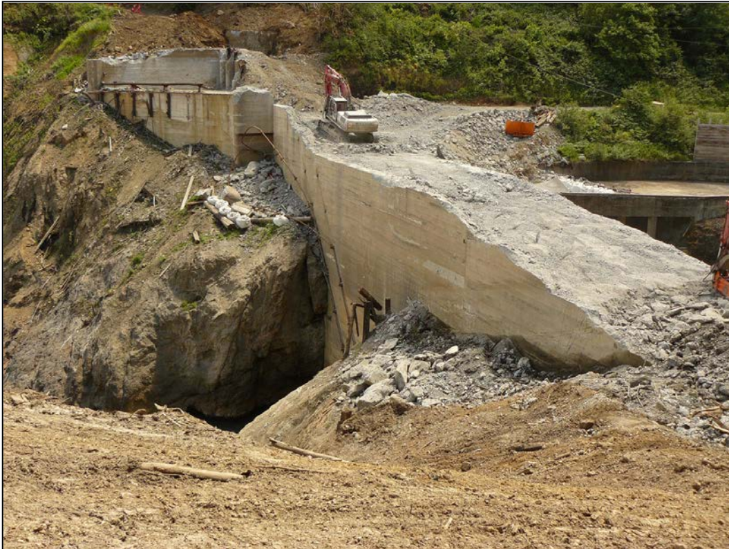
Figure 240: Condit Dam Removal, July 2012 (Courtesy of Andy Maser and Steve Stampfli)
