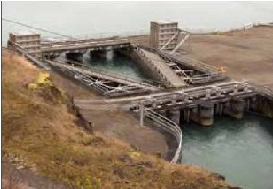
Figure 95: One of two Mayfield Dam Downstream Migrant Collection Louver Arrays (Photo Courtesy of Tacoma Power)
