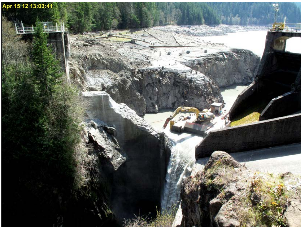
Figure 227: Glines Canyon Dam – April 15, 2012 (Courtesy of the NPS)
