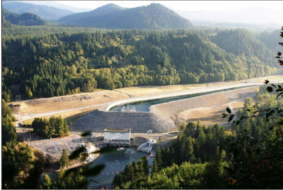
Figure 104: Swift No. 2 Powerhouse (Courtesy of Cowlitz PUD)
