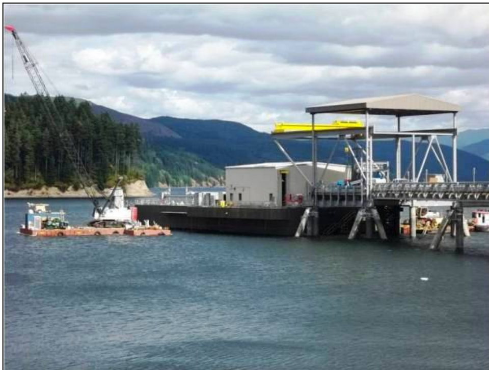
Figure 111: Swift FSC and Access Trestle (Courtesy of PacifiCorp)
