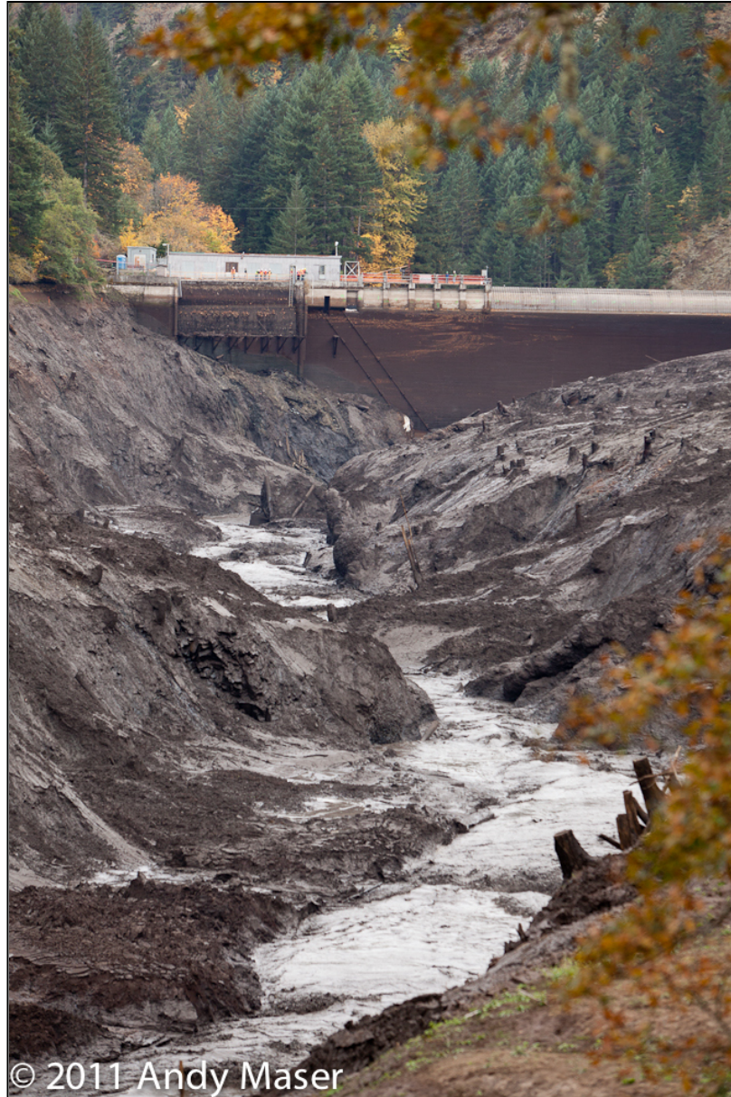
Figure 235: Northwestern Reservoir and Condit Dam after the breach (Courtesy of Andy Maser and Steve Stampfli)
