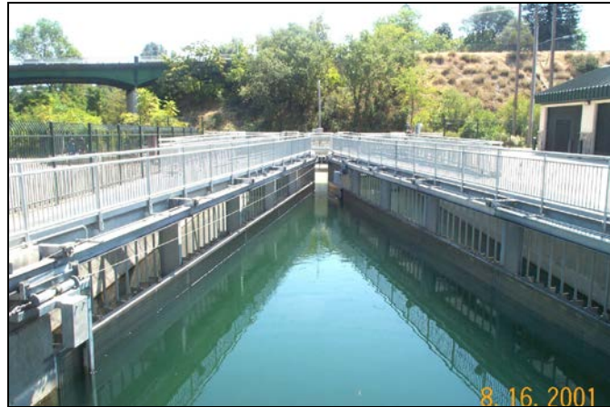
Figure 45: ACID Diversion Vertical Flat-plate Fish Screen in “V” Formation, Sacramento River, CA (CA Dept. of Water Resources)
