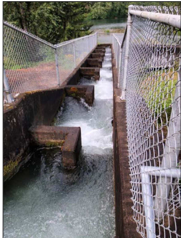
Figure 88: Cowlitz Salmon Hatchery separator ladder (CA Dept. of Water Resources)
