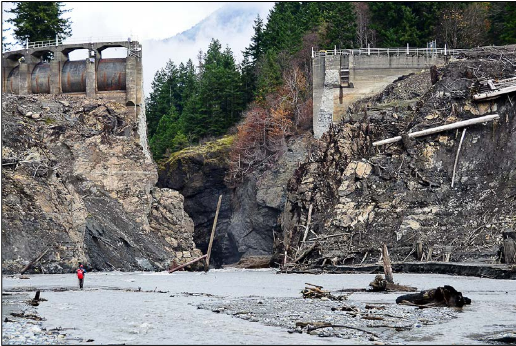
Figure 230: Glines Canyon Dam from Upstream - November 6, 2012 (Courtesy of Brian Cluer, NMFS)
