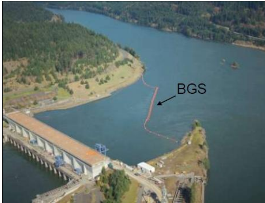
Figure 121: Behavioral Guidance System in the second powerhouse forebay (source: USACE)
