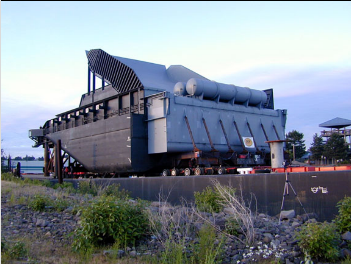
Figure 136: Removable Spillway Weir, before installation at Lower Granite Dam (source: USACE)
