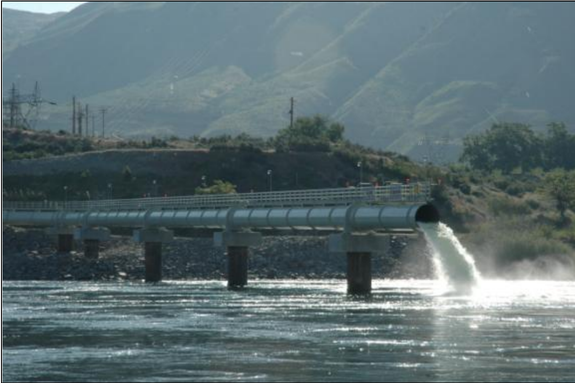
Figure 127: Close-up of Rocky Reach juvenile bypass system tailrace exit (Courtesy of Chelan County PUD)
