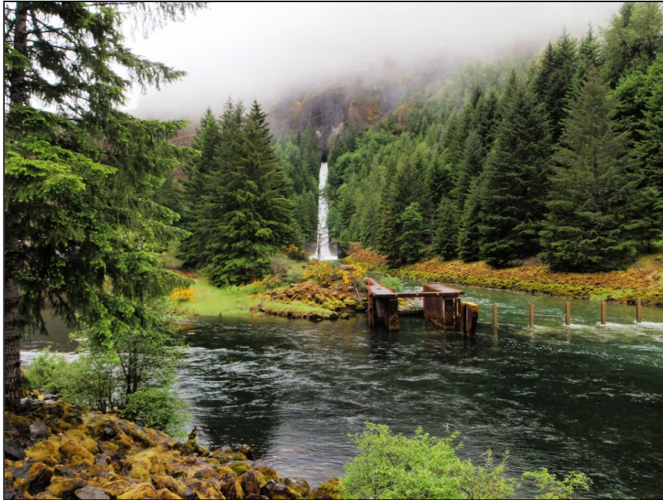
Figure 145: Regulating Outlet (CA Dept. of Water Resources)
