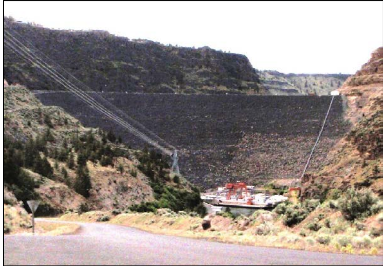
Figure 177: Round Butte Dam and Hatchery (CA Dept. of Water Resources)
