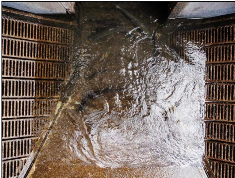
Figure 181: Pelton Trap Brail Pool (CA Dept. of Water Resources)
