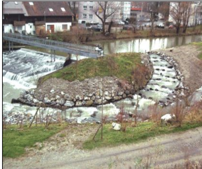
Figure 22: Nature-like bypass channel (Photo courtesy of Rolf-Jurgen Gebler)
