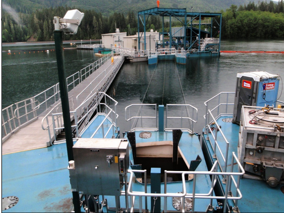
Figure 76: Upper Baker Dam FSC fish barge and tank (right) – photo taken from dam (CA Dept. of Water Resources)
