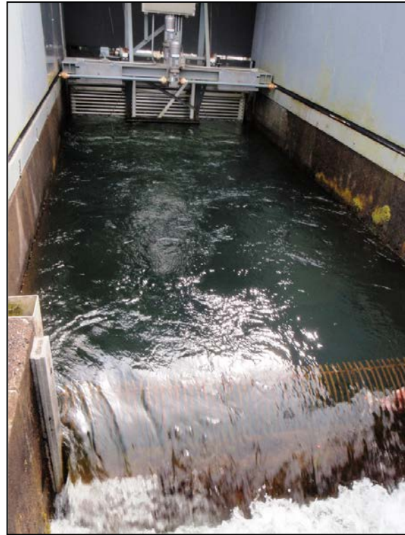
Figure 89: Cowlitz Salmon Hatchery finger weir and holding pool (CA Dept. of Water Resources)
