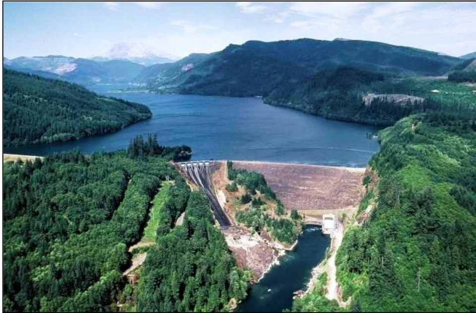
Figure 106: Yale Dam (Courtesy of Low Impact Hydropower Institute)
