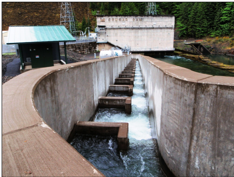
Figure 14: Half Ice Harbor Fishway at Cougar Dam on the South Fork McKenzie River (CA Dept. of Water Resources)
