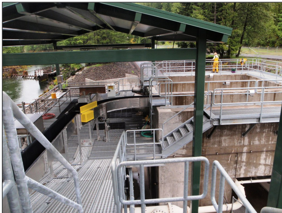
Figure 153: Sorting Area and Post-Sort Pools (CA Dept. of Water Resources)
