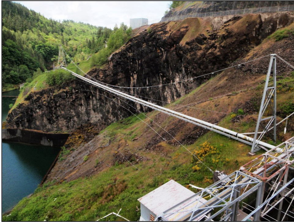
Figure 101: Mayfield Downstream Migrant Bypass Pipe (CA Dept. of Water Resources)
