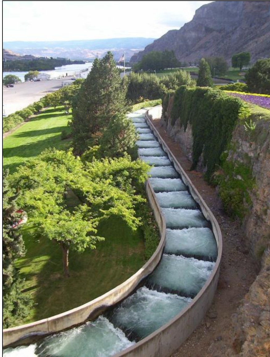
Figure 123: Pool and weir fish ladder at Rocky Reach Dam (This file is licensed under the Creative Commons Attribution ShareAlike 3.0 License. Photo taken by: Garrett Fitzgerald)
