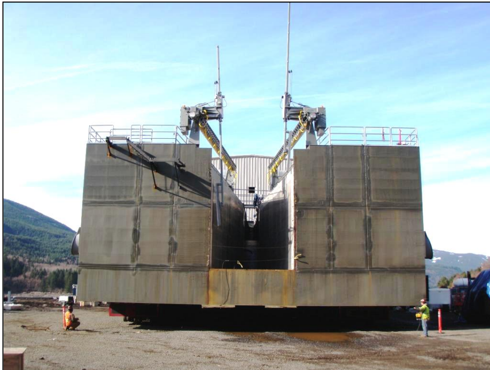
Figure 108: Swift FSC Fish Entrance (Courtesy of PacifiCorp)
