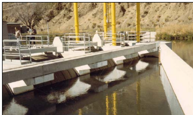
Figure 42: Roza Diversion Dam Drum Screens, Yakima River, WA (USBR)
