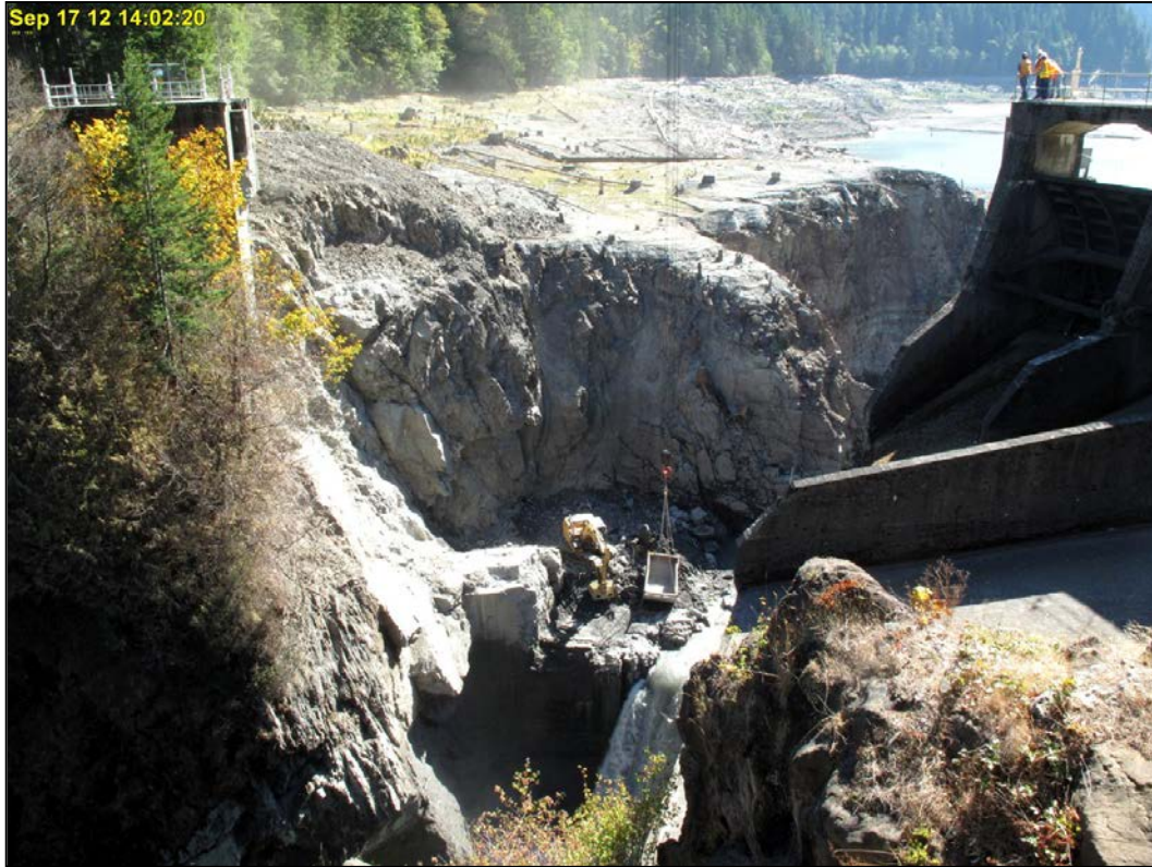
Figure 228: Glines Canyon Dam – September 17, 2012 (Courtesy of the NPS)
