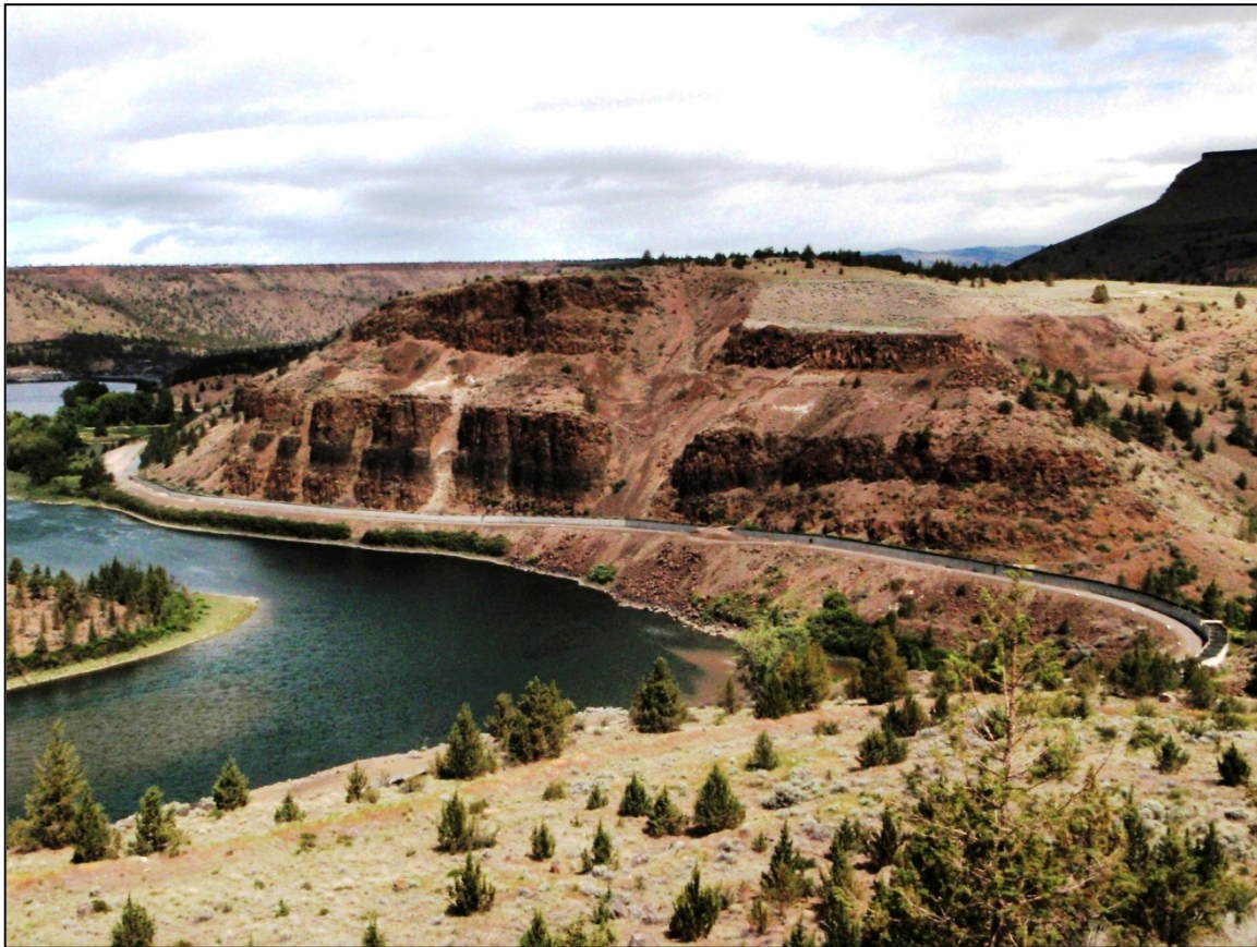
Figure 184: Pelton Fish Ladder along Reregulating Reservoir (CA Dept. of Water Resources)
