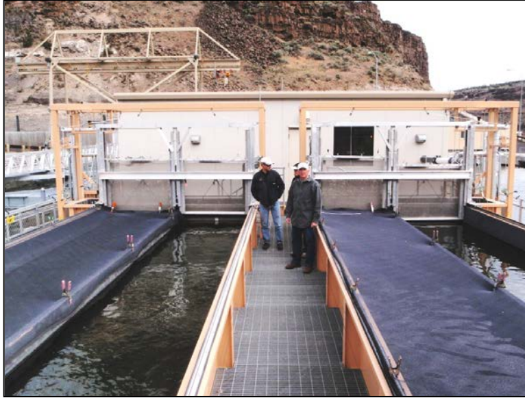
Figure 197: Holding Raceways with Fish Processing Building in Background (CA Dept. of Water Resources)
