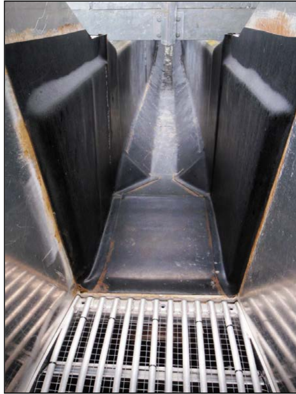
Figure 152: False Weir and Flume to Sorting Area (CA Dept. of Water Resources)
