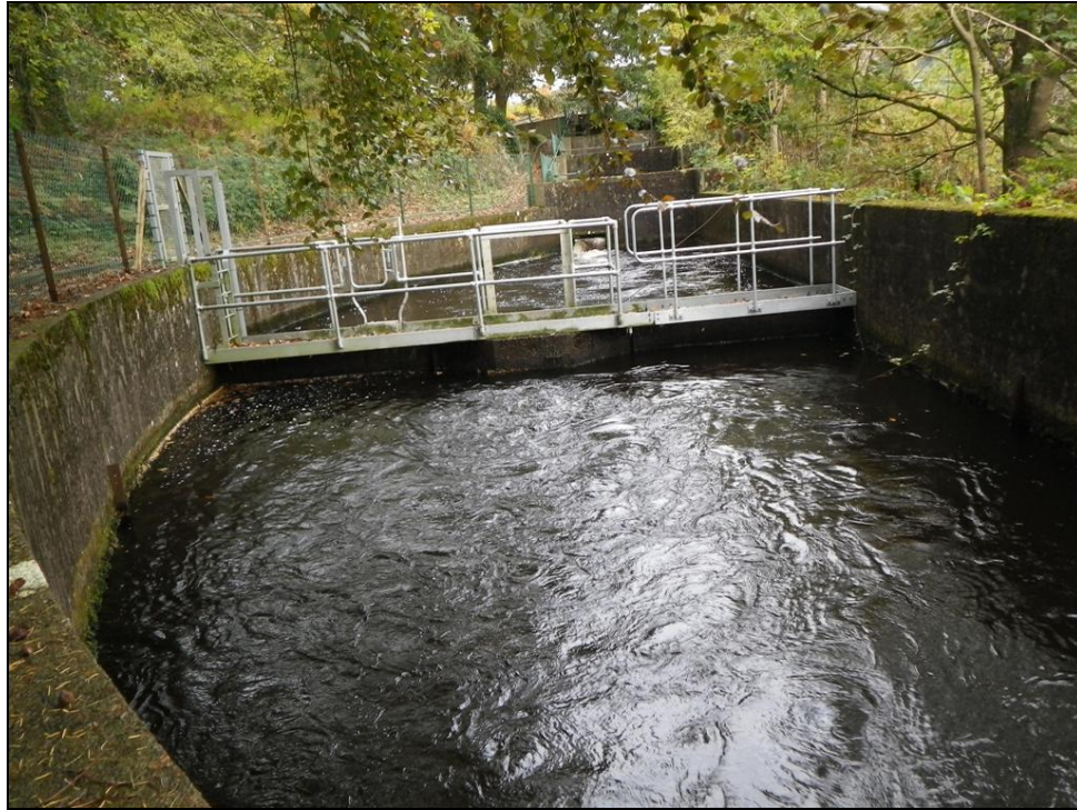
Figure 210. Weir in resting pool 3 – with submerged orifice and fish counter tunnel (Courtesy of Galloway Fisheries Trust)
