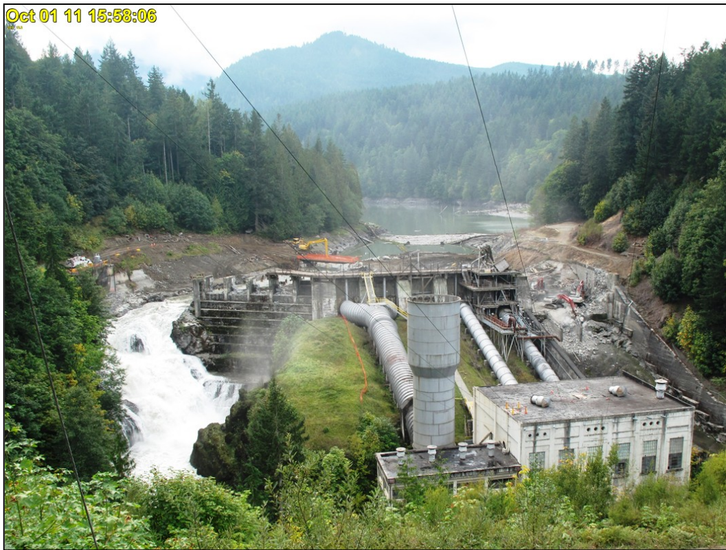
Figure 219: Elwha Dam – October 1, 2011 (Courtesy of the NPS)
