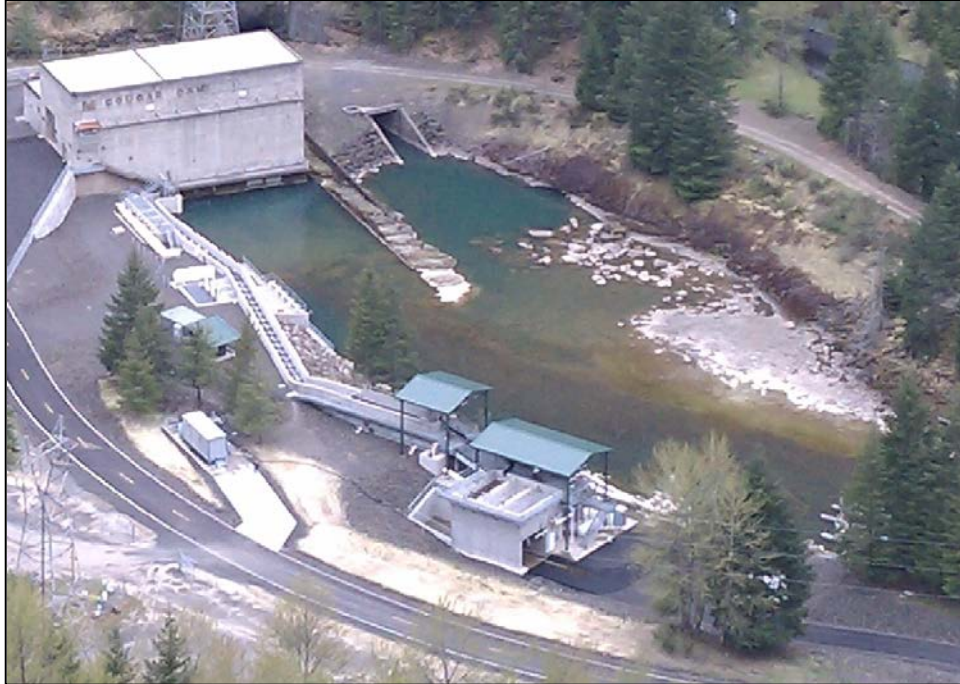
Figure 148: Overview of the Adult Collection Facility (Courtesy of USGS)
