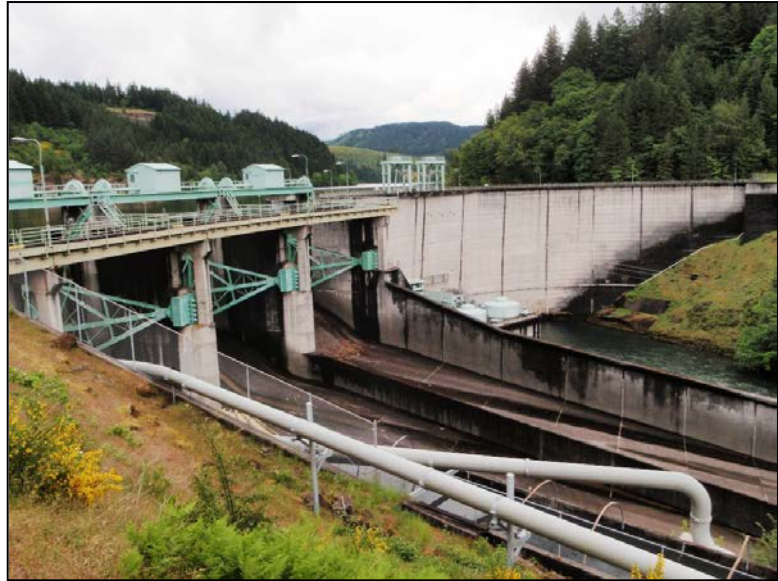
Figure 161: North Fork Dam (CA Dept. of Water Resources)
