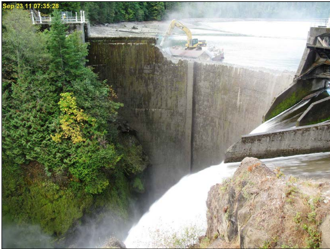
Figure 224: Glines Canyon Dam - September 23, 2011 (Courtesy of the NPS)
