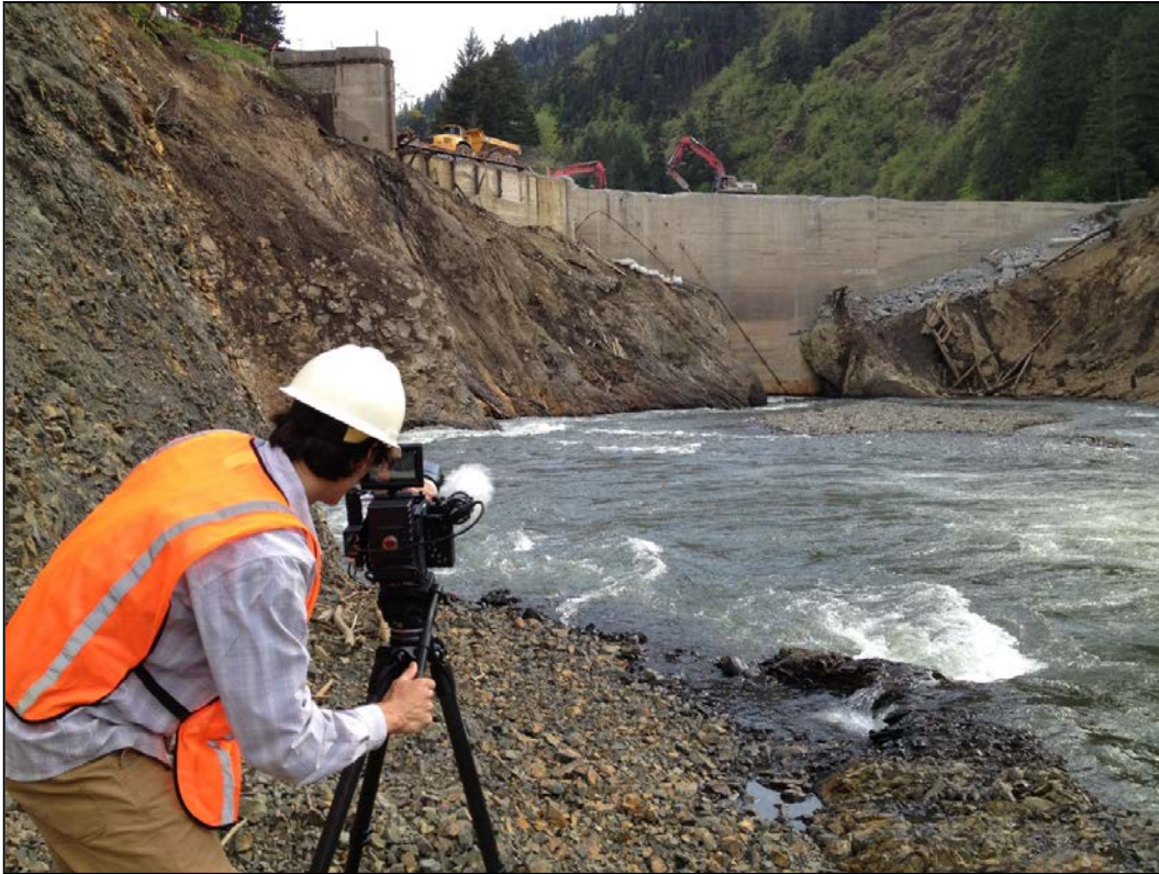
Figure 238: Condit Dam Removal, May 2012 (Courtesy of Andy Maser and Steve Stampfli)
