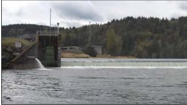
Figure 83: Barrier Dam with Downstream Migrant Outfall Pipe (Photo Courtesy of Tacoma Power)
