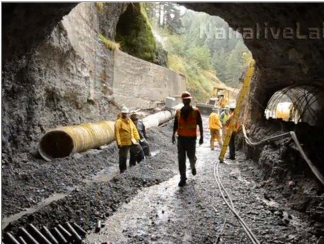
Figure 233: Breach Tunnel (Courtesy of Narrative Lab)
