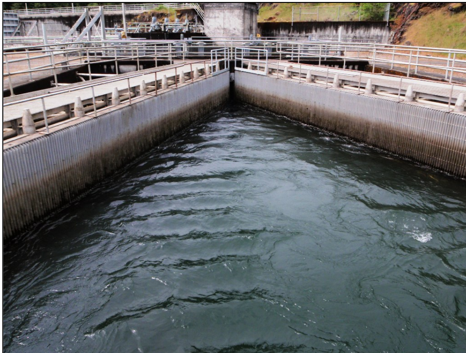
Figure 96: Mayfield Downstream Migrant Collection Louver Array (CA Dept. of Water Resources)
