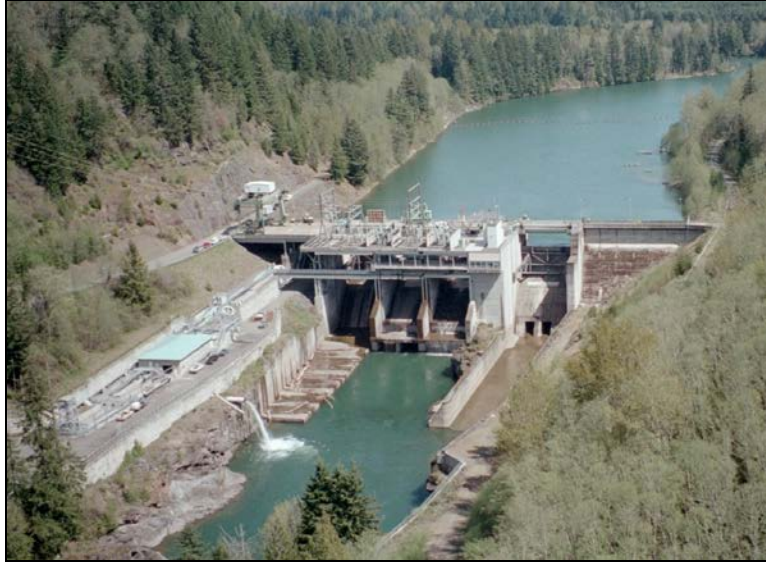
Figure 84: Cowlitz Falls Dam with Fish Facility on Left Side of Photo (Photo Courtesy of Lewis County Public Utility District)
