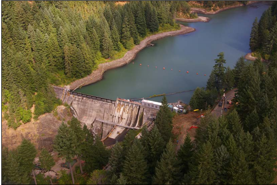
Figure 232: Condit Dam (Courtesy of PacifiCorp)
