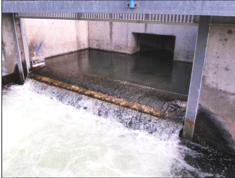
Figure 180: Pelton Trap Finger Weir and Entrance Pool (CA Dept. of Water Resources)
