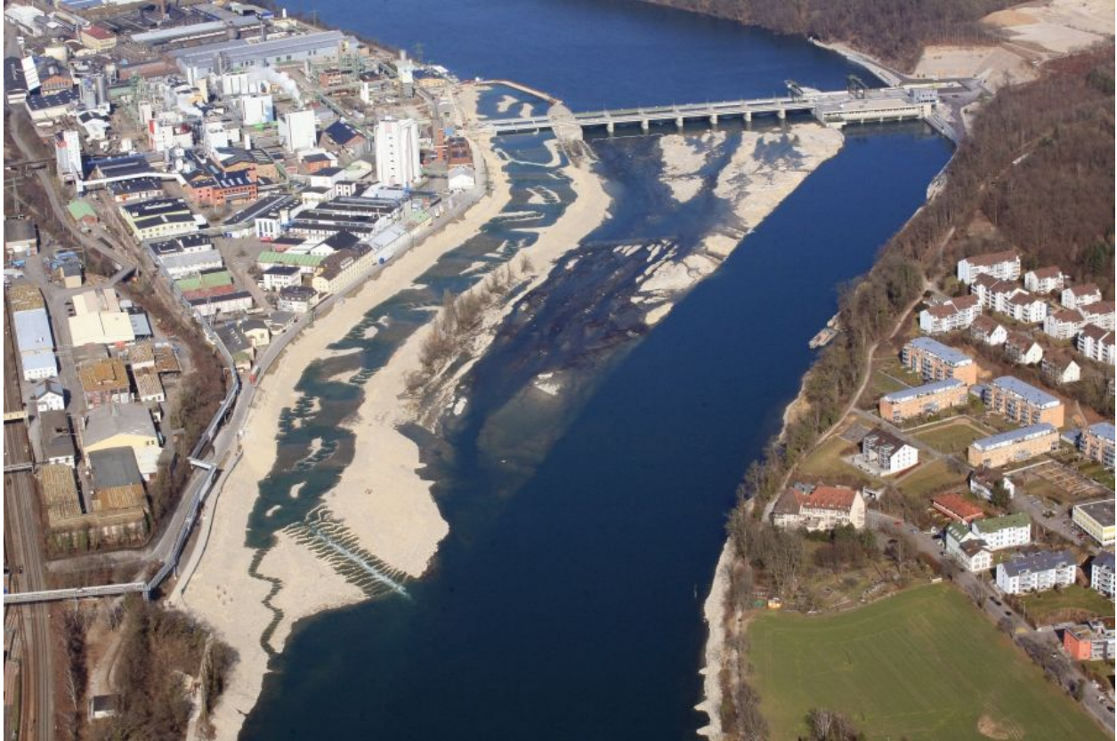
Figure 23: Aerial view of the nature-like bypass channel at the Rheinfelden Power Station on the Rhine River (Courtesy of Rolf-Jurgen Gebler)
