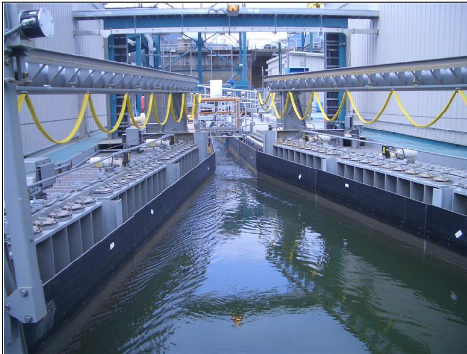
Figure 74: Upper Baker Dam FSC primary fish screens (NOAA Fisheries)
