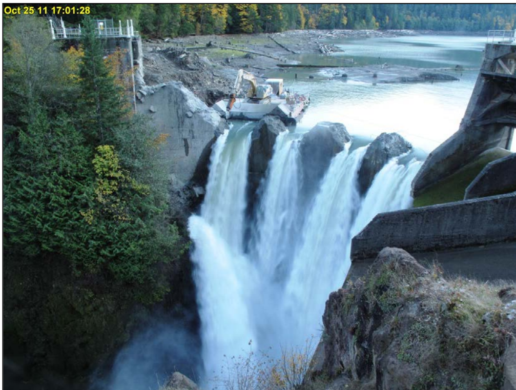
Figure 225: Glines Canyon Dam - October 25, 2011 (Courtesy of the NPS)
