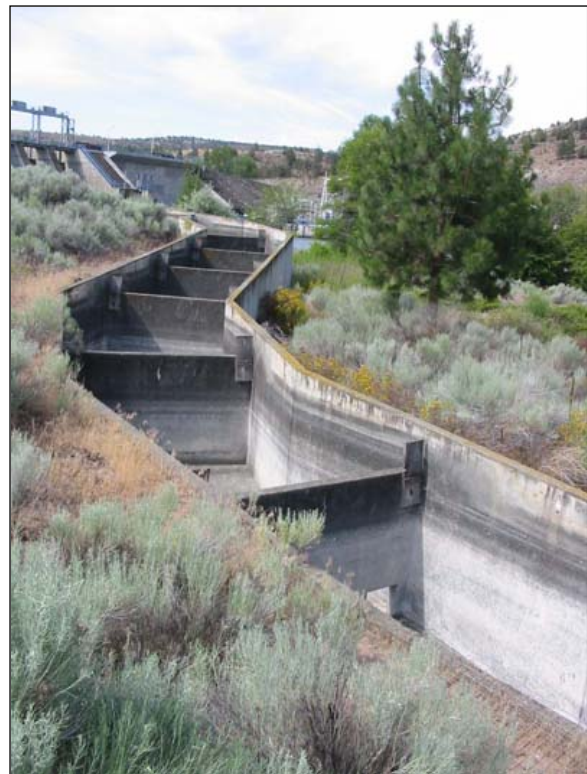
Figure 183: The Lower End of the Pelton Fish Ladder (Courtesy of PGE)
