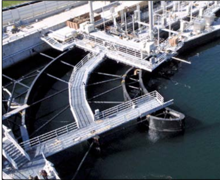
Figure 124: Twin entrances to juvenile bypass surface collector, forebay Rocky Reach Dam (Courtesy of Chelan County PUD)
