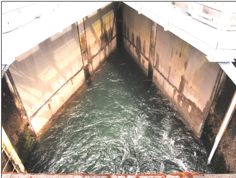
Figure 98: Mayfield Downstream Migrant Collection Facility Secondary Screens (CA Dept. of Water Resources)
