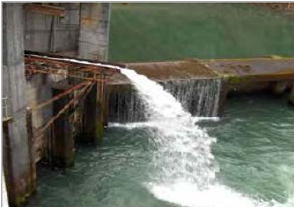
Figure 102: Downstream Migrant Release Flume (Photo Courtesy of Tacoma Power)
