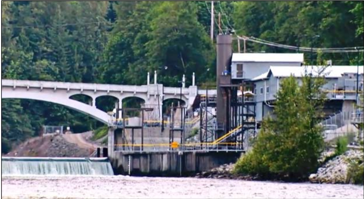
Figure 31: Adult fish trap and lock on the Baker River, Washington (Courtesy of Puget Sound Energy)
