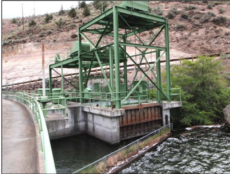
Figure 187: Pelton Skimmer (CA Dept. of Water Resources)
