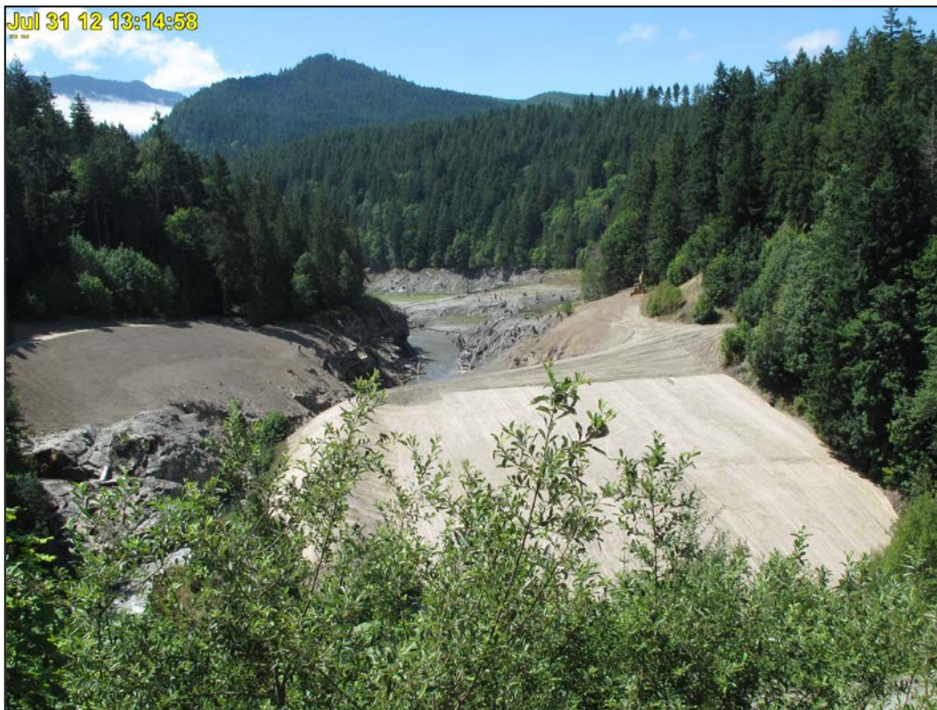
Figure 223: Elwha Dam Site after Removal - July 31, 2012 (Courtesy of the NPS)
