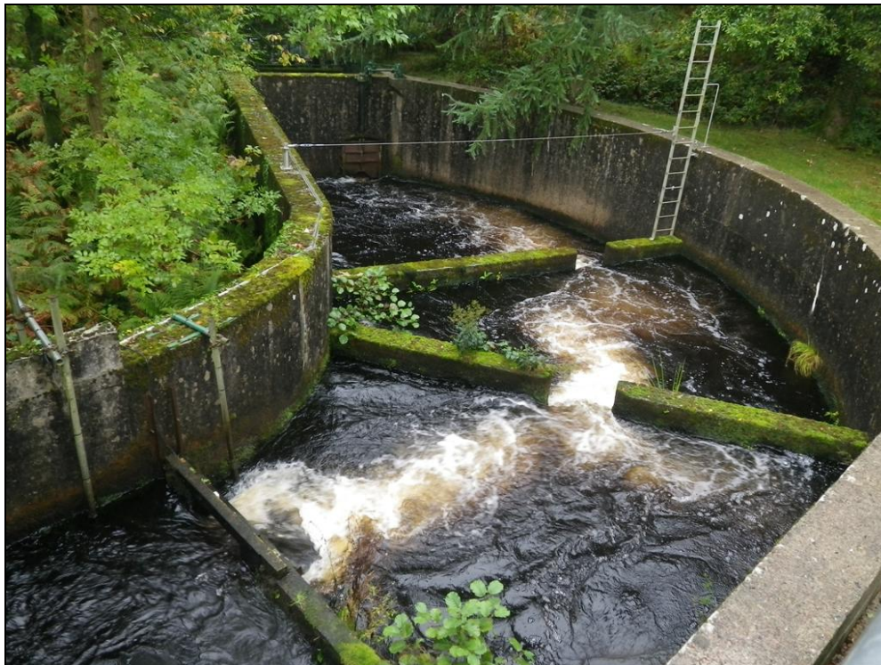
Figure 211. Section 5 of the fish ladder (Courtesy of Galloway Fisheries Trust)
