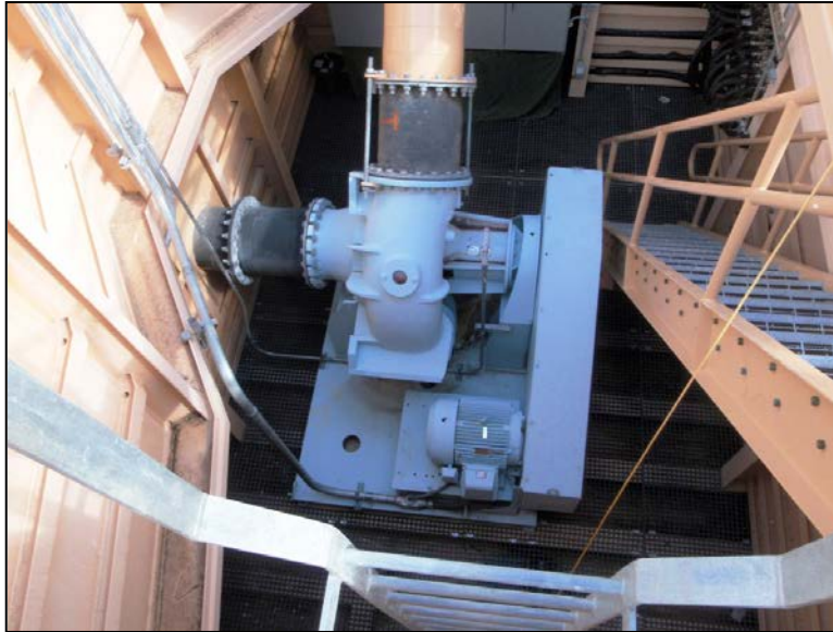
Figure 195: Hidrostal Fish Pump (CA Dept. of Water Resources)
