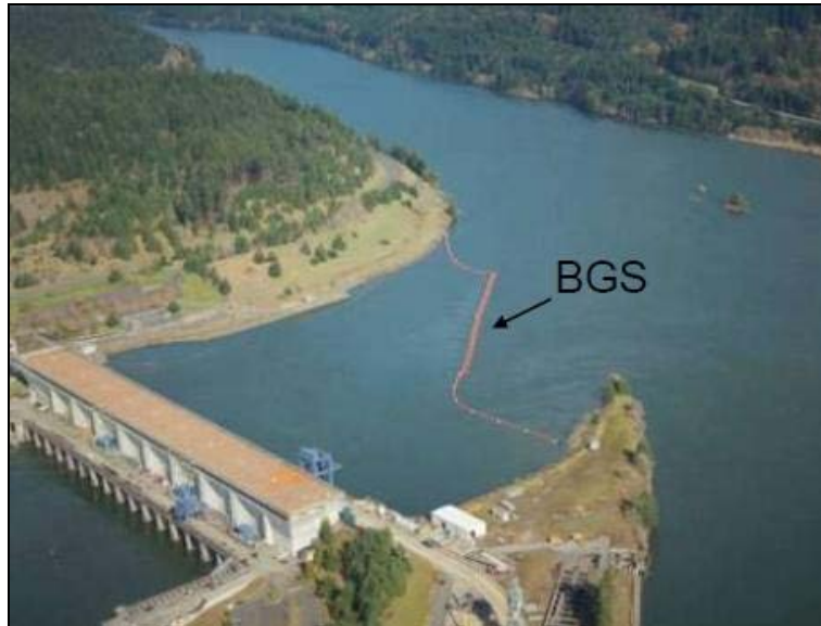
Figure 54: Behavioral Guidance System at Bonneville Dam (Courtesy USACOE)
