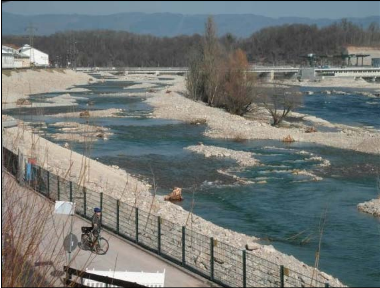
Figure 24: Nature-like bypass channel at the Rheinfelden Power Station on the Rhine River (Courtesy of Rolf-Jurgen Gebler)
