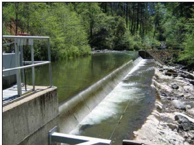
Figure 49: Montgomery Creek Coanda Fish Screen (Wahl 2003)
