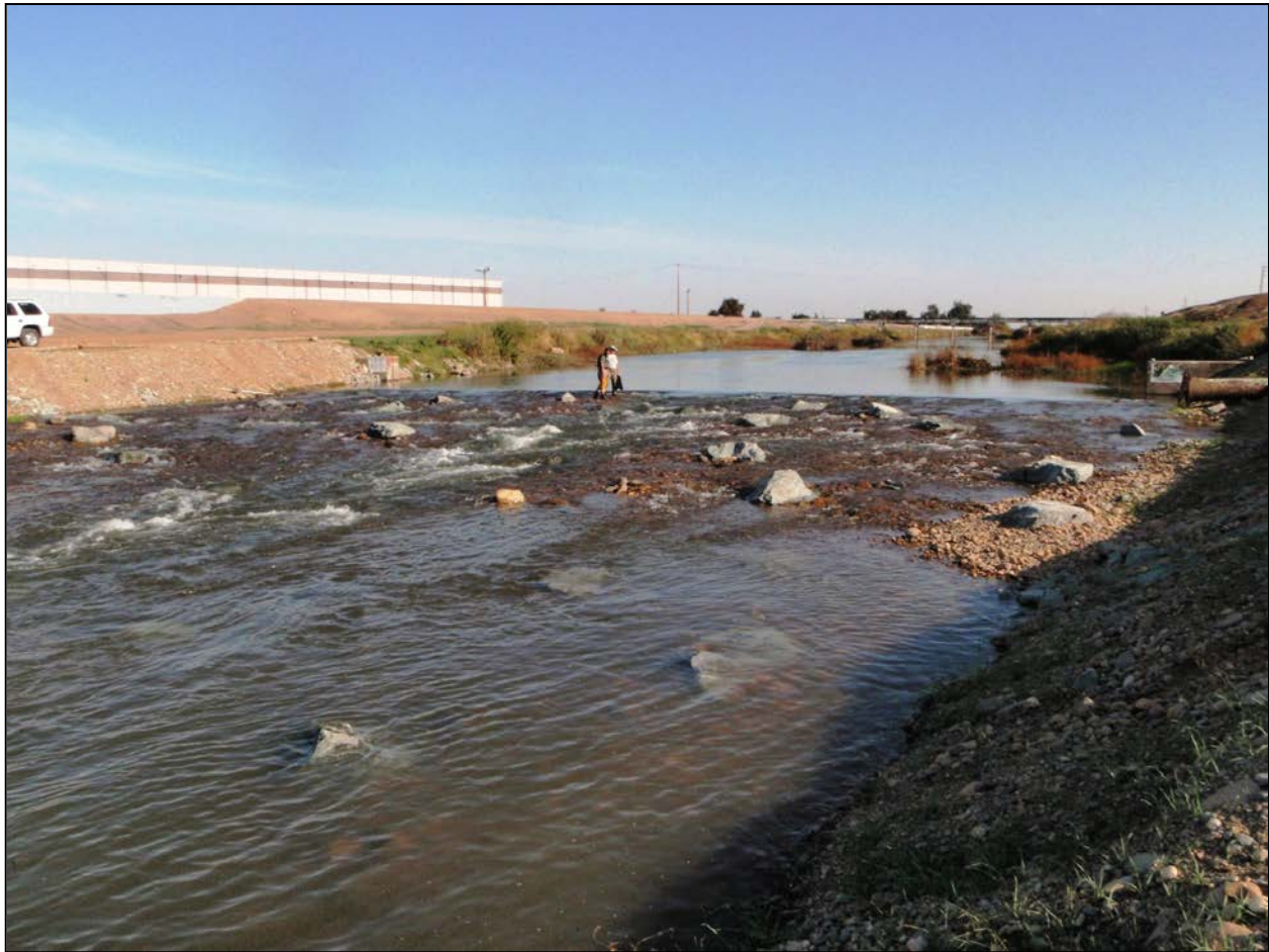
Figure 25: Rock ramp roughened channel at the Budiselich Flashboard Dam site in the Stockton Diverting Canal, Calaveras River System (CA Dept. of Water Resources)
