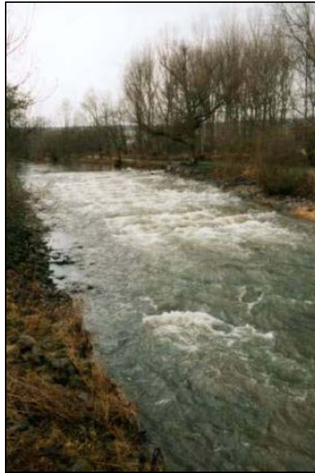
Figure 20: Full width nature-like (rock ramp) fishway (Photo by Uli Dumont in Wildman et al 2002)
