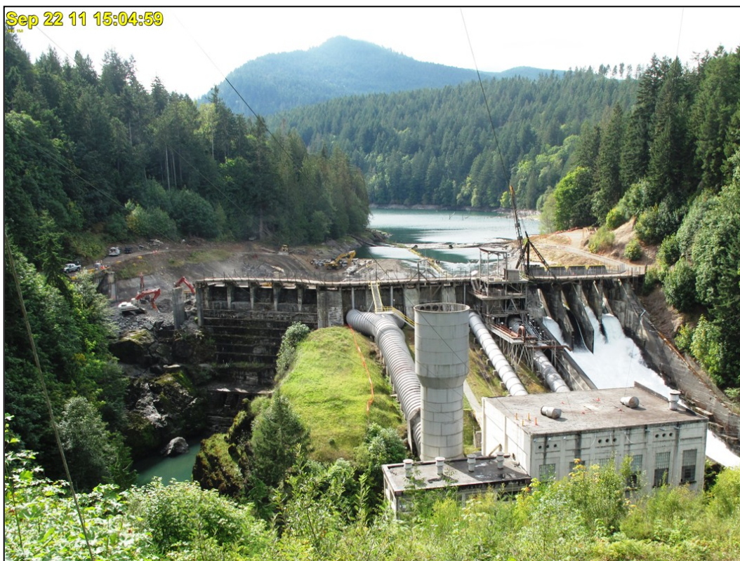
Figure 218: Elwha Dam - September 22, 2011 (Courtesy of the NPS)
