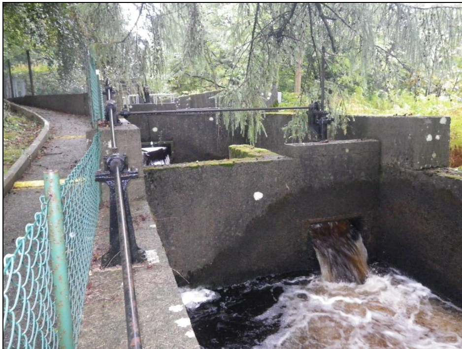
Figure 207. Orifice section – upstream view (Courtesy of Galloway Fisheries Trust)
