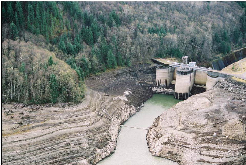
Figure 113: Swift Intake Channel at Low Reservoir Elevation (Courtesy of PacifiCorp)
