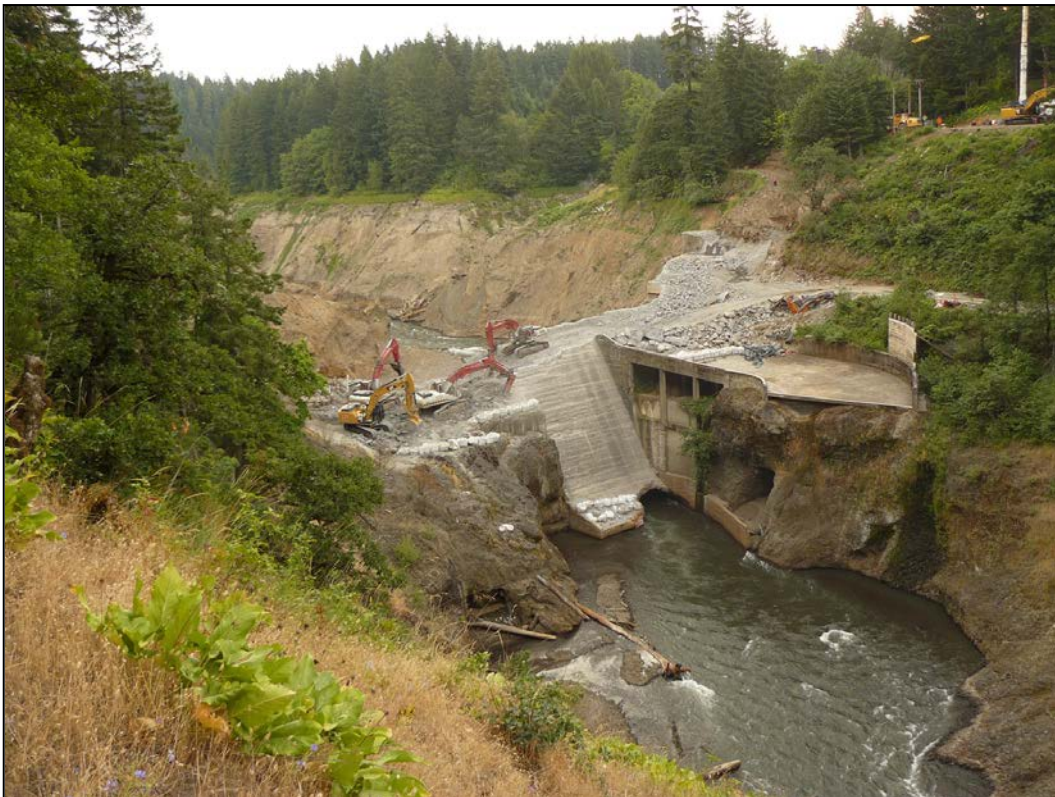
Figure 239: Condit Dam Removal, July 2012 (Courtesy of Andy Maser and Steve Stampfli)
