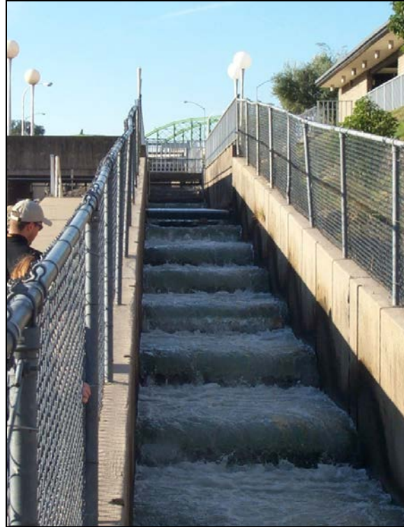
Figure 11: Pool and Weir Fishway at the Feather River Fish Hatchery, California (CA Department of Water Resources)
