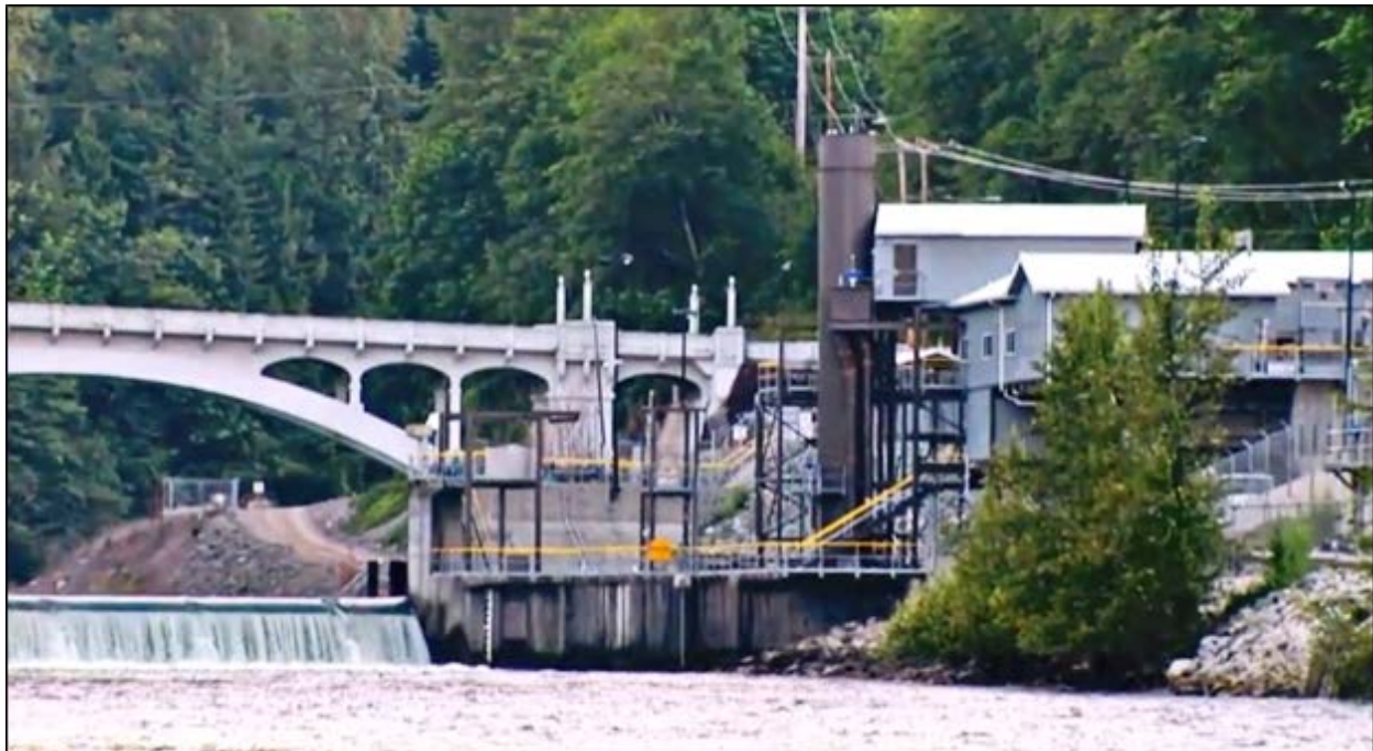
Figure 63. Adult fish trap facility, below Lower Baker Dam (Courtesy of PSE)
