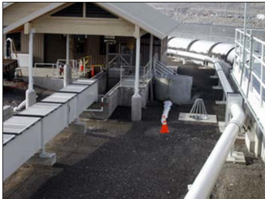
Figure 125: Rocky Reach juvenile bypass sampling facility: fish condition and run-timing is monitored. Smolts are also collected for acoustic tagging in survival studies. (Courtesy of Chelan County PUD)
