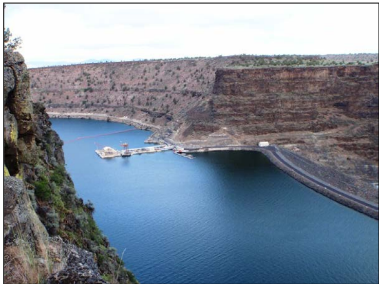
Figure 178: Round Butte Dam and the Downstream Fish Collection Facility (CA Dept. of Water Resources)
