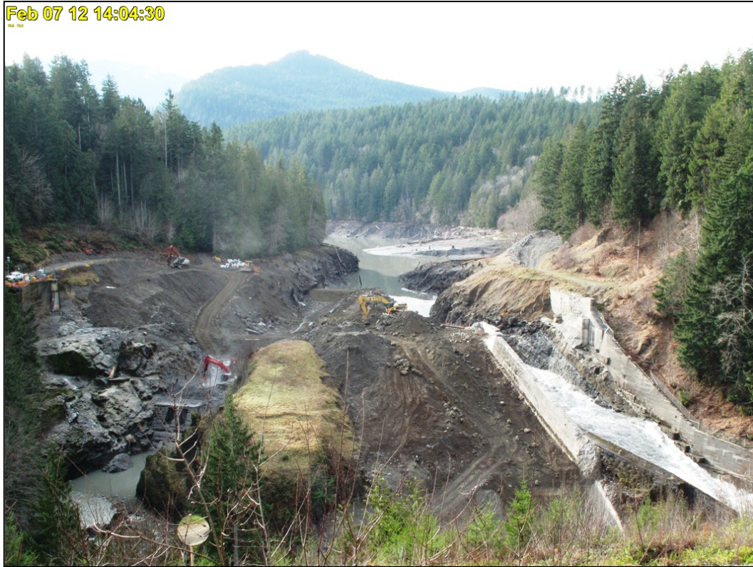
Figure 221: Elwha Dam – February 7, 2012 (Courtesy of the NPS)
