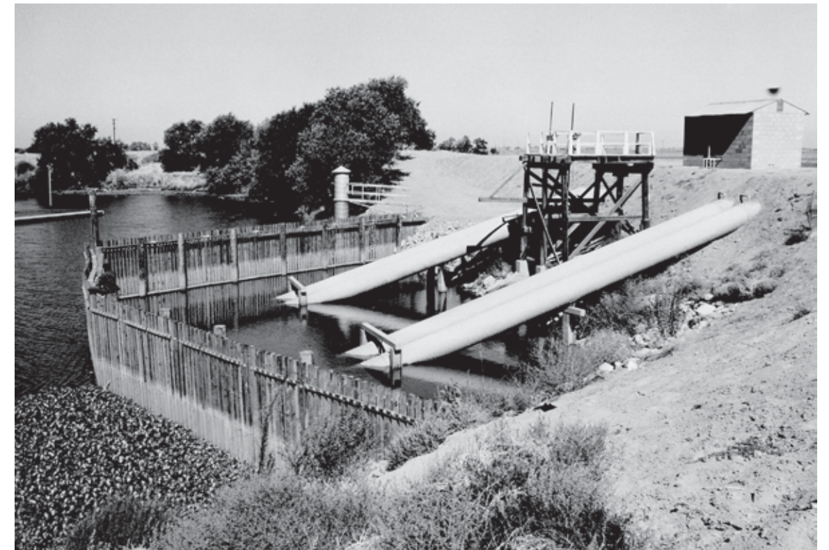
Siphons at Tom Paine Slough, installed as part of a settlement contract to improve water quality in a portion of the South Delta Water Agency.
