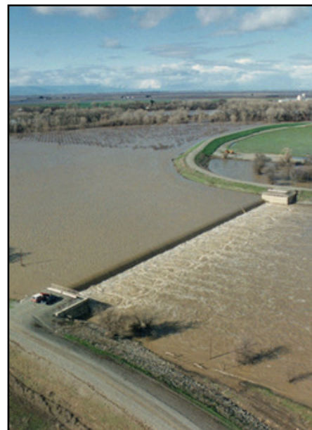
Moulton Weir spills water into the Butte Basin
