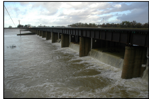
The Sacramento Weir is the only weir that requires manual operation for flow release
