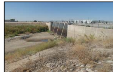
The Chowchilla Canal Bypass Control Structure is an SPFC facility
