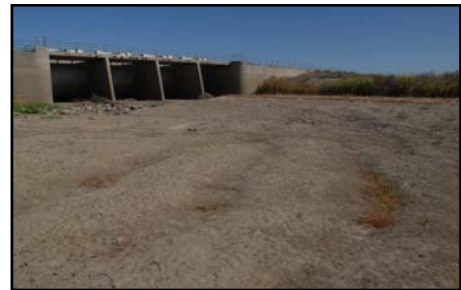
Levees line the channel downstream from the Chowchilla Bypass Control Structure
