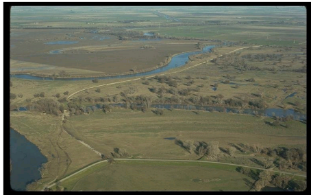
The Sacramento River and the joint channel for the Sutter Bypass and Feather River join at the Fremont Weir
