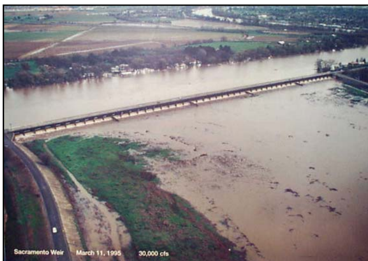
The Sacramento Weir provided flood protection for the City of Sacramento in 1995
