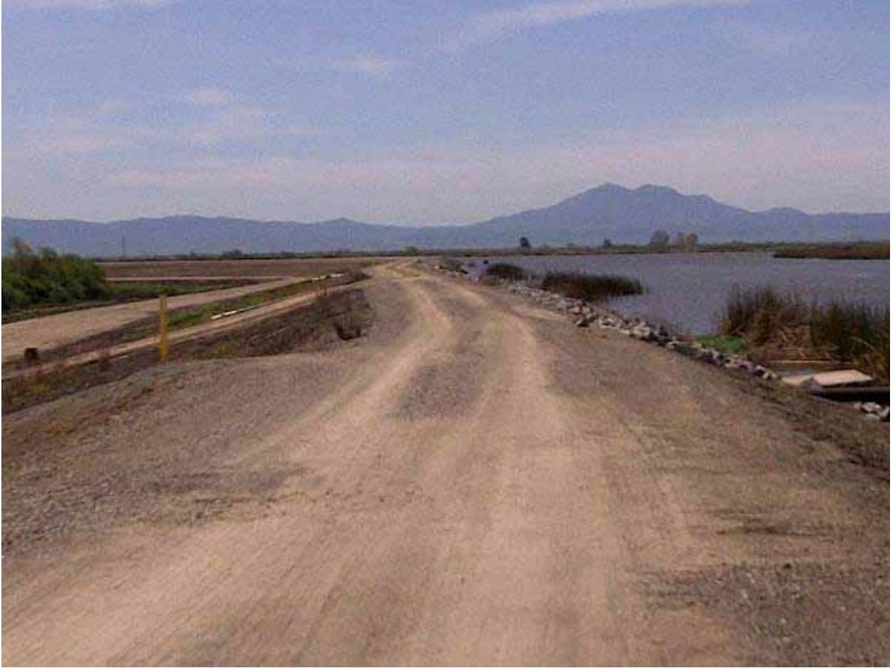
Figure C-9 - McDonald Island, showing PL 85-99 berm on landside
