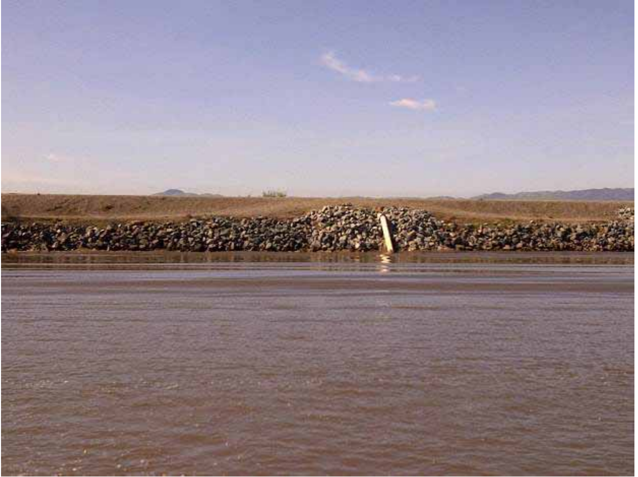
Figure C-8 - Byron Tract, showing stepped seismically-resistant levee
