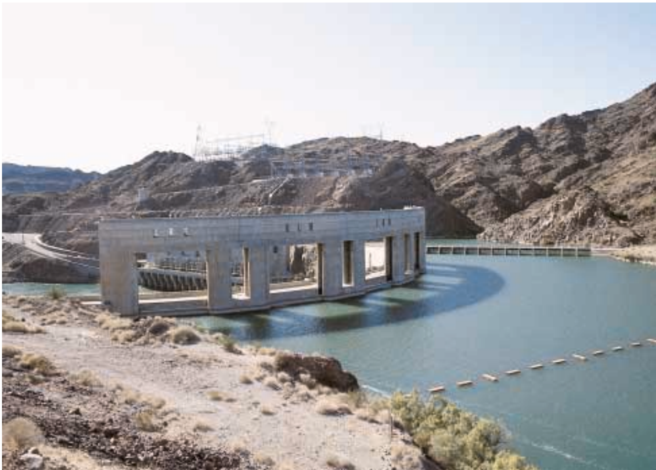
USBR's Parker Dam on the Colorado River impounds Lake Havasu, the point of diversion for MWD's Colorado River Aqueduct. Since the CRA is the only facility linking the river with urbanized coastal Southern California, its conveyance capacity is the limiting factor on the coastal region's use of river water.
