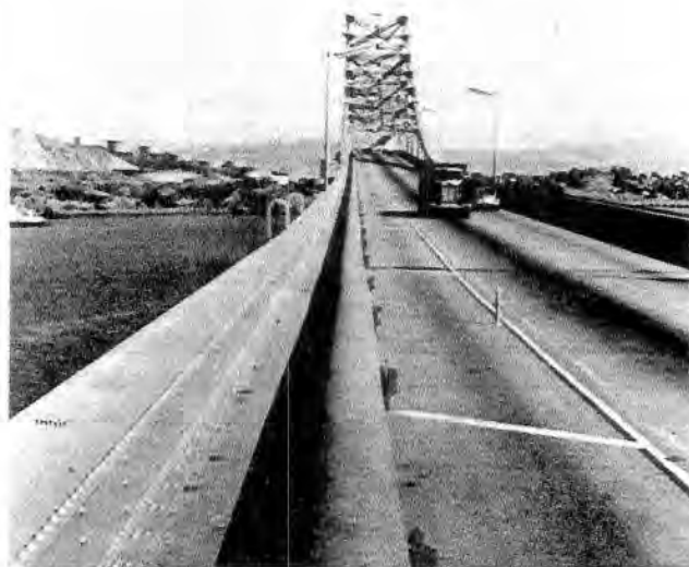
41. Water for Marin County. Shown here is the emergency pipeline on the Richmond-San Rafael Bridge as it approaches San Rafael. (Marin MWD photo.)
