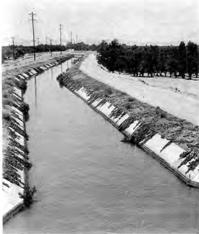
12. A transfusion for Contra Costa. Shown is the Contra Costa Canal, the major source of water for industrial, agricultural, and urban uses in Contra Costa County. With the construction of the barriers at Rock and Indian Sloughs and the Middle River facilities, CCCWD received higher quality water than would have otherwise been possible.
