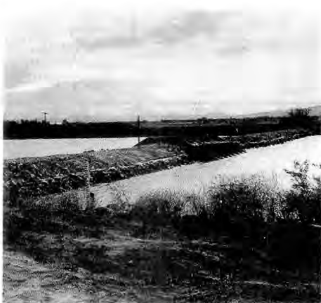
6. Guardian of the South Delta. The Dutch Slough barrier, west of Antioch, prevented the inflow of salt water and kept the salt content at an acceptable level.
