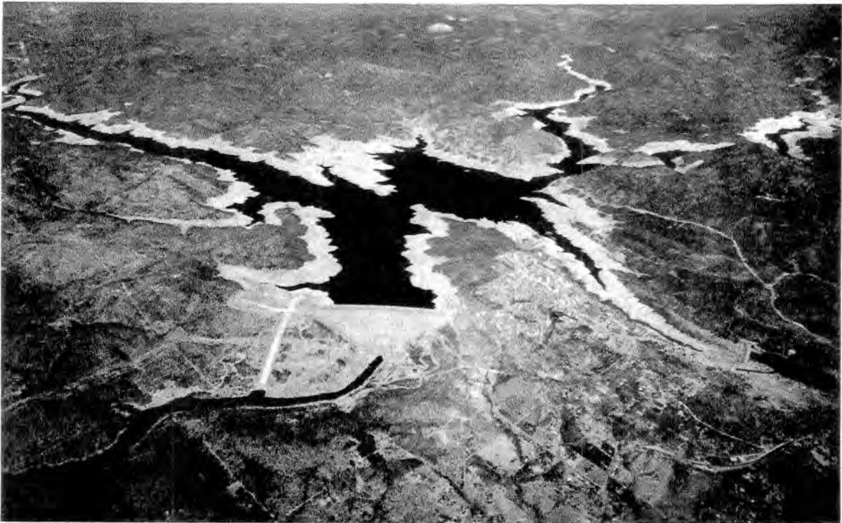
7. Low on reserves. Lake Oroville as it appeared on September 30, 1977. Storage on that date was only 1 100 cubic hectometres (915,000 acre-feet), or about one-fourth of capacity. Lake Oroville reached its lowest point on September 7.
