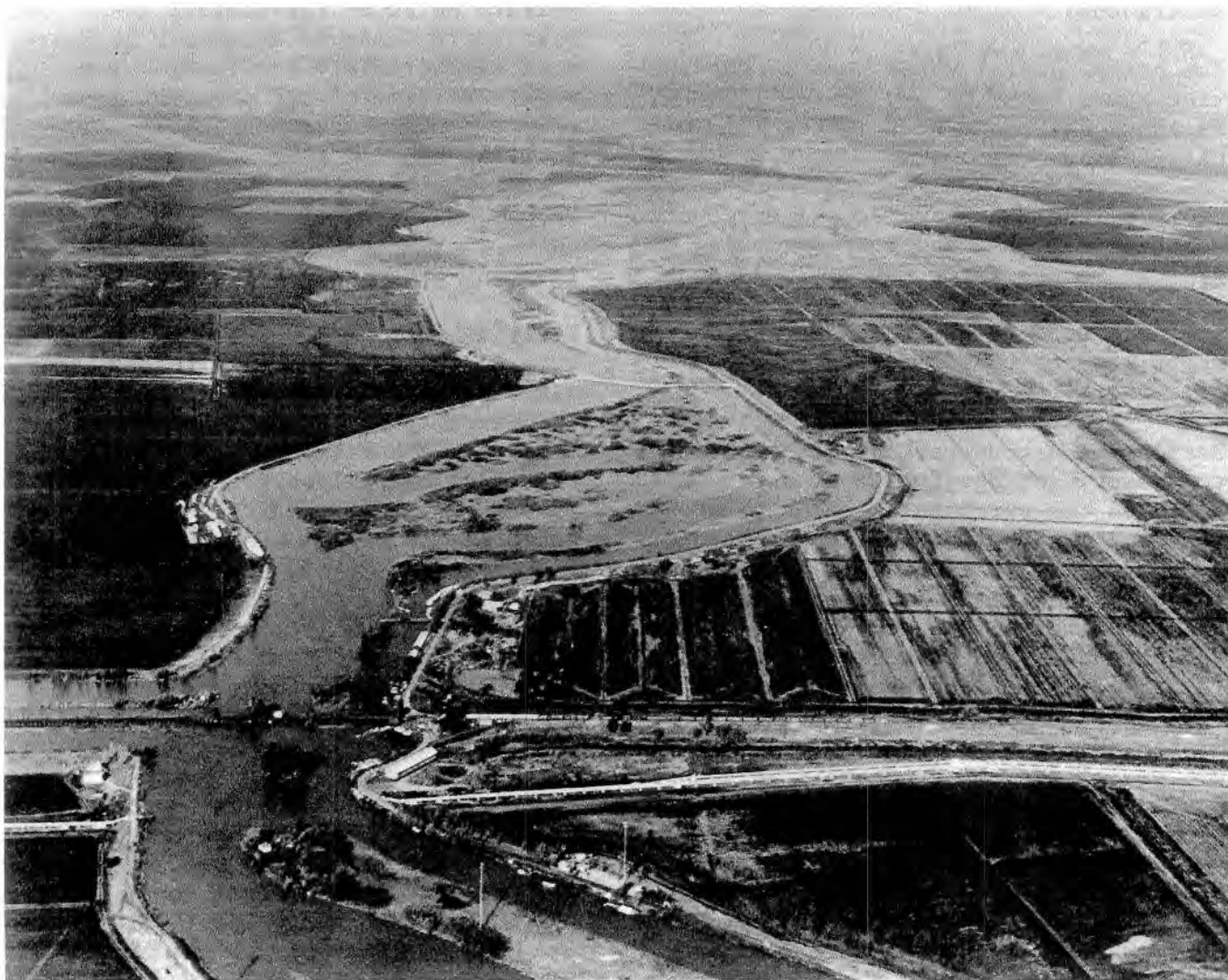
8. Before the drought. The Mokelumme Aqueduct is seen crossing Middle River. This photograph was taken before the drought necessitated the construction of the Middle River pumping facilities.
