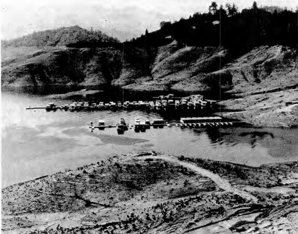
23. The traveling marinas. As levels at Shasta Lake began to drop, these floating docks had to be moved farther downslope. At the right is the temporary road leading down to the disappearing reservoir.
