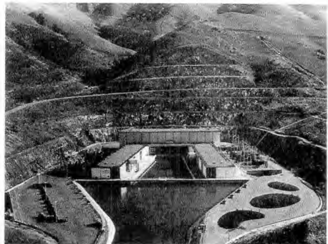
54. Water for the cities. The A. D. Edmonston Pumping Plant near Bakersfield, where water from the California Aqueduct is lifted over the Tehachapi Mountains for delivery to Southern California, saw little use in 1977 as the available supplies were shifted to Northern and Central California instead. 1978 will see a return to more normal deliveries.
