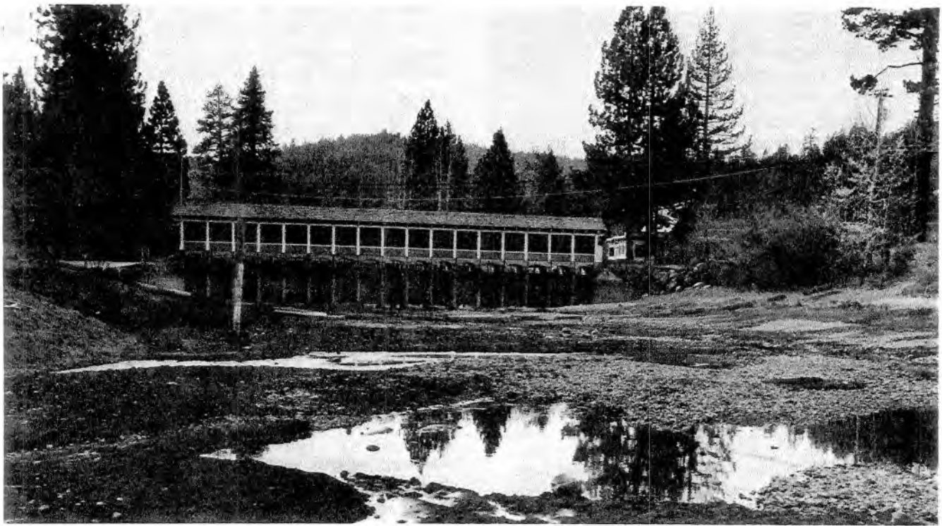
33. The Lake Tahoe Outlet near Tahoe City. The Truckee River ceased flowing when the level at Lake Tahoe dipped below that of the outlet. The photographer was standing within Lake Tahoe's ordinary pool.
