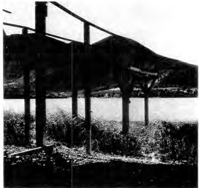
22. A useless mooring. This boat pier on the northeast shore of Clear Lake is typical of the many boat launching facilities rendered unusable as a result of the drought.
