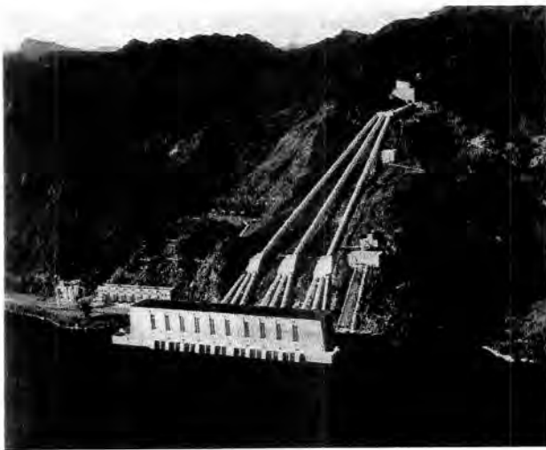
9. Helping hands across the State. The Colorado Aqueduct Pumping Plant, shown here pumping from Lake Havasu into the Colorado River Aqueduct for delivery to MWD, was the keystone in the complicated water exchange which allowed additional water to be retained for use in Northern and Central California.
