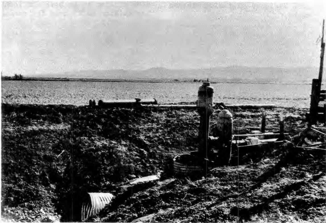
35. Drought aid to farmers. During the drought, several programs were made available to implement soil and water conservation practices. The photographs show a newly lined ditch (to prevent seepage loss) and a tailwater return system. (Soil Conservation Service photos.)
