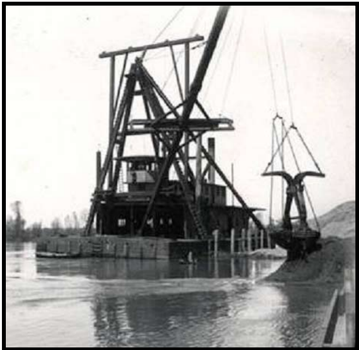
Sidedraft clamshell dredger constructing levees using alluvial soil. 6
