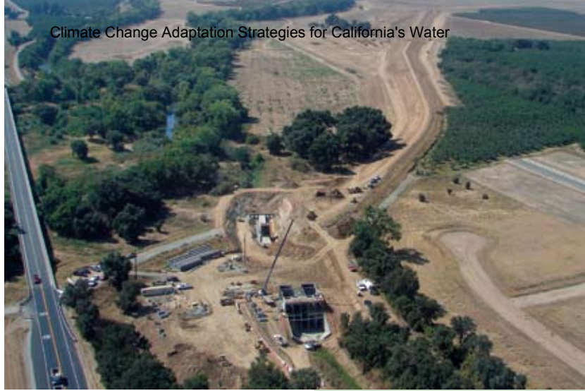
Setback levee being constructed near Bear River
