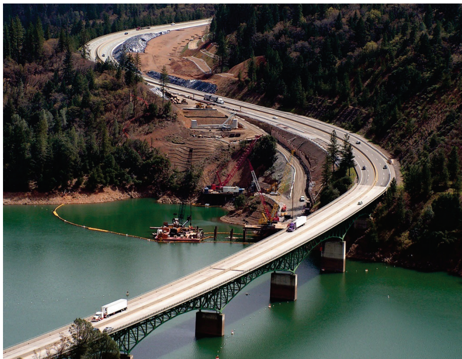
Photo 1 Caltrans I-5 Antlers Bridge Realignment Project on Shasta Lake
