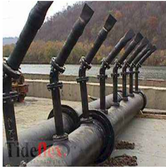
An example of a multiport diffuser, which rapidly mixes, disperses, and dilutes brine. This is seen as an acceptable method of brine discharge by the Water Board.
