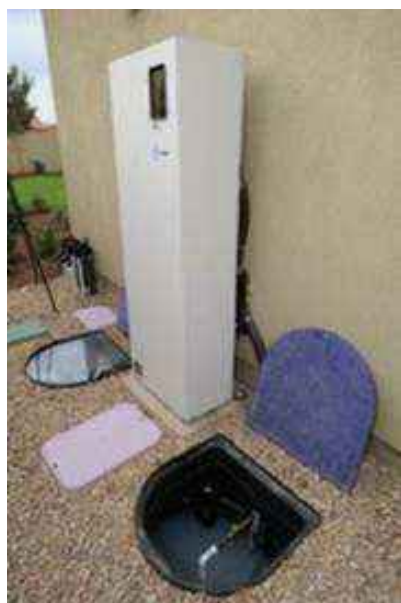
An onsite reuse system installed in a family home.
