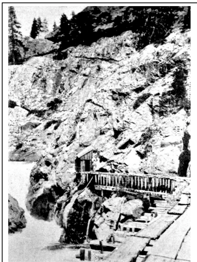
Figure B9. Trestled wood box flume, head of South Yuba Ditch (PG&E Archives)
