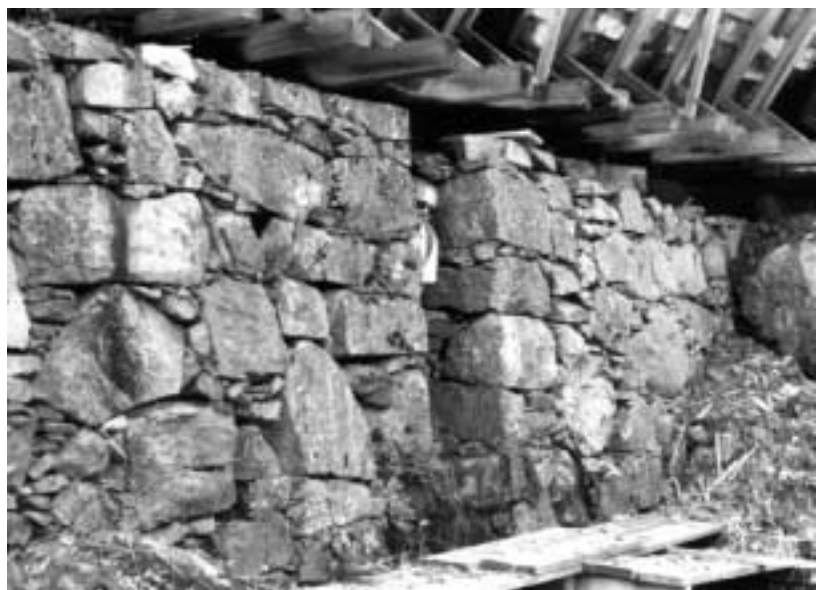
Figure 19. El Dorado Canal bench flume showing side drainage notch (JRP Collection)
