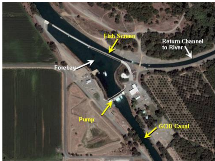
Glenn-Colusa Irrigation District Canal Intake Source: DWR, 2007
