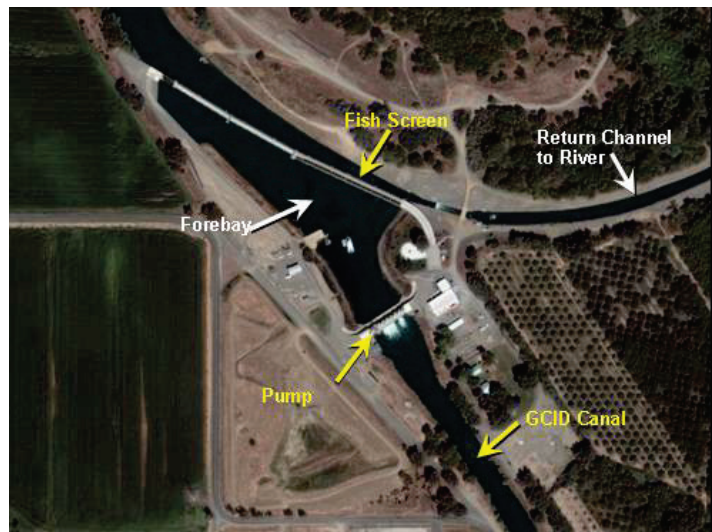
Glenn-Colusa Irrigation District Canal Intake
