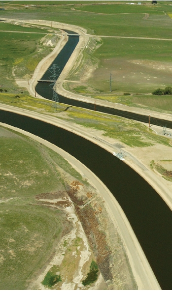
California Aqueduct and Delta Mendota Canal intertie
